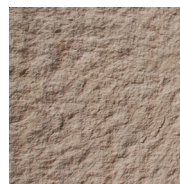
Wall Finish to Cutting Rough textured finished concrete.
