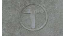
Fibreglass Telecom marking
