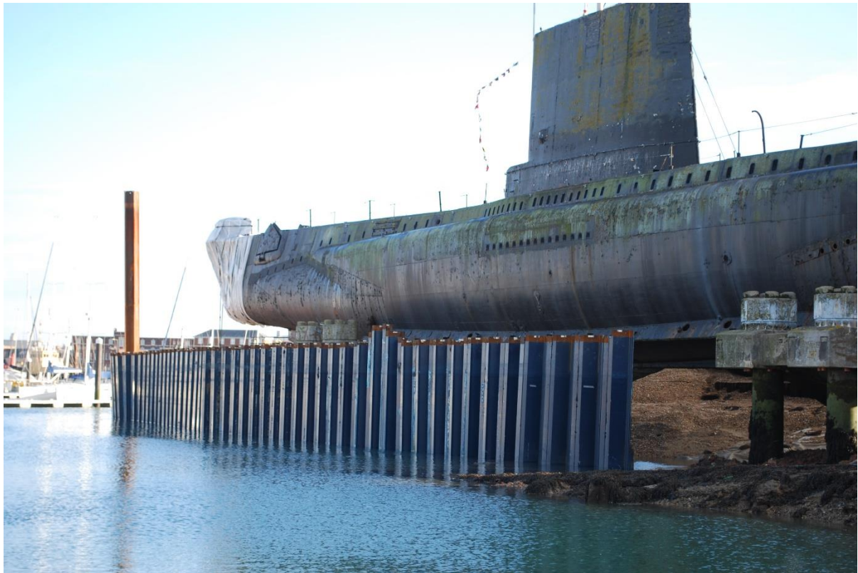
Cofferdamn Under Construction in 2010-11 (prior to restoration of submarine)
