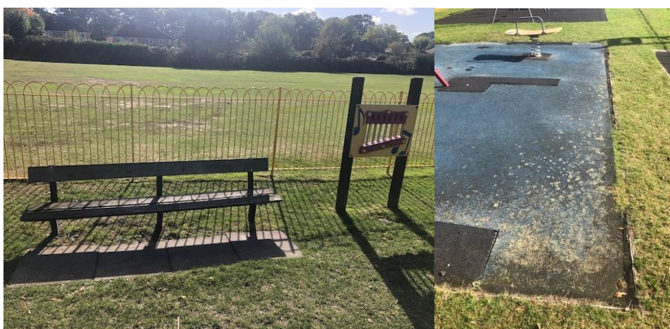
2 x Benches and Play Panel to be removed and disposed of. All surfacing, edging and board springer shown on photo above (right) to be removed and disposed of – some areas have exposed foundations that need to be cut below surface level as will any new removals.
