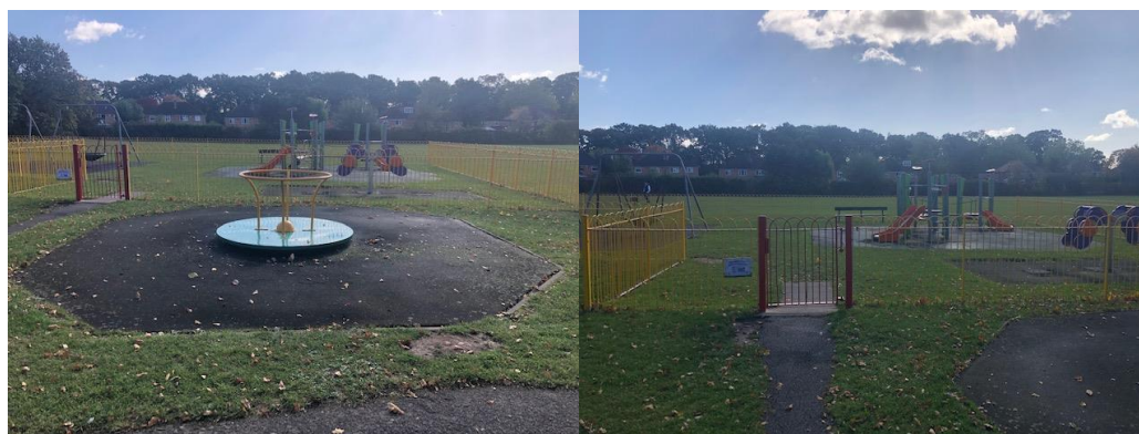
Surfacing under roundabout to be replace with new wetpour and possibly stone base. New pathway to connect existing tarmac path to gate (photo on right).
