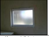
Presumed to contain asbestos unless proven otherwise. No access within the window and frame and sill due to damage limitations. As agreed with Sarah Willsher on site. Applies to all 15 windows within the Changing Facilities building.
