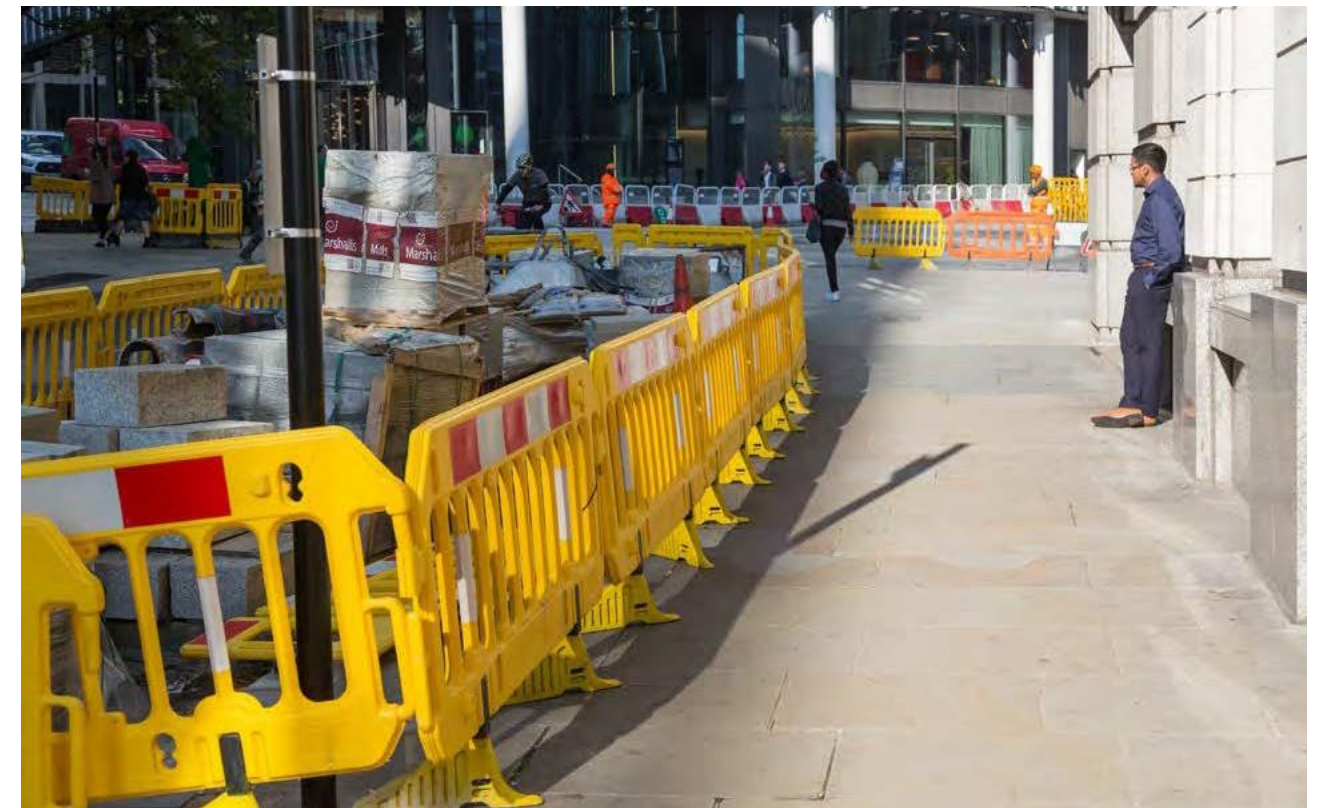
Good practice: tidy, correctly assembled and well-maintained barrier
