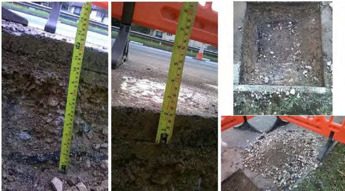
Example 1 – Trial pit construction close up showing legible measurement and construction layers
