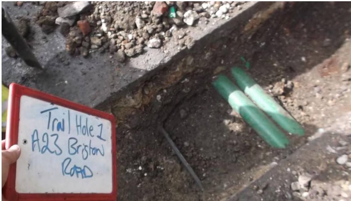
Figure 2 – Trial pit construction and stats services
