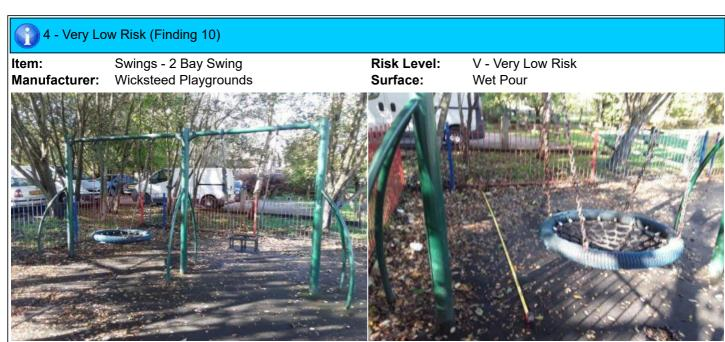
**Finding:** BS EN 1176 requires an additional 0.5m of unobstructed space at each end of the swing surfacing area. This is a relatively low risk finding and no remedial action is recommended at this point. **Action:** Monitor - No remedial work recommended work recommended area.
