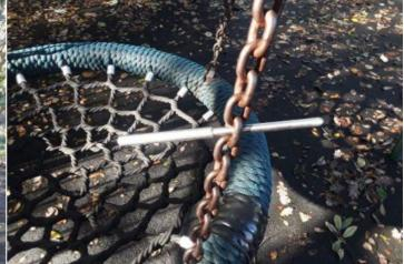
**Finding:** The chain openings are in excess of the 8.6mm as **Action:** Monitor - No remedial work recommended recommended by BS EN 1176
