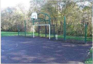
Finding: There is/are finger entrapments in the framework Action: Monitor - No remedial work recommended and the item fails to meet the requirements of BS EN 15312 Clause 4.4.2.2 Entrapment of fingers
