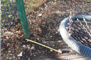
**Finding:** The seats are too close to the frame as defined in BS EN 1176 Part 2; this is a low risk failure and no remedial action is required
