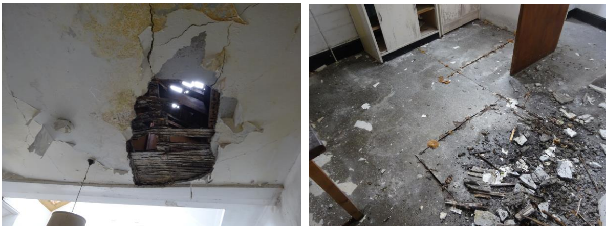
22. Collapsed ceiling to kitchen on left – dry rot affected flooring to right
