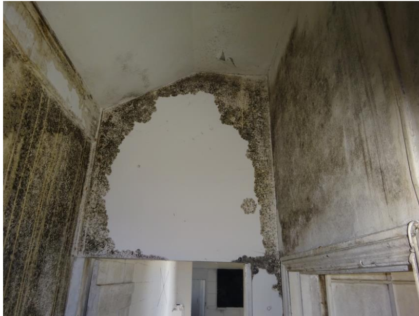
24. Mould to stairwell walling due to water ingress.
