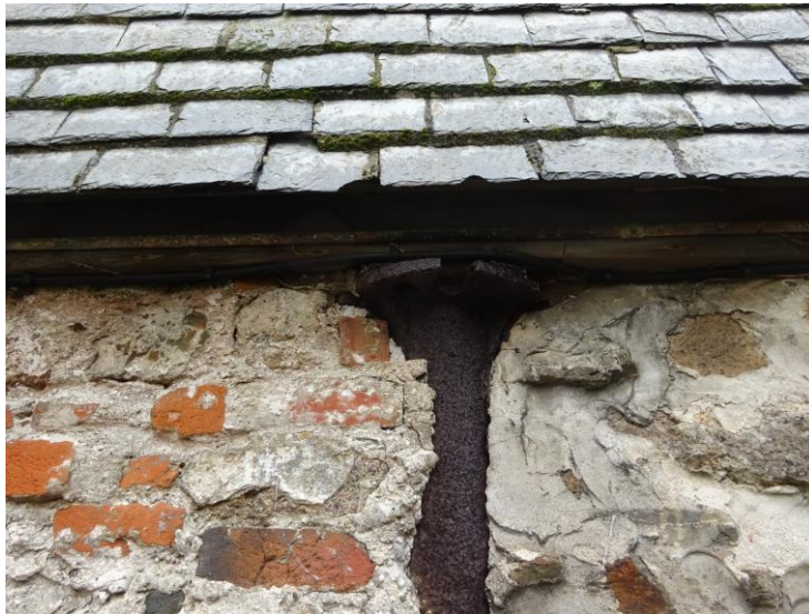
11. Embedded iron columns with masonry infill between.
