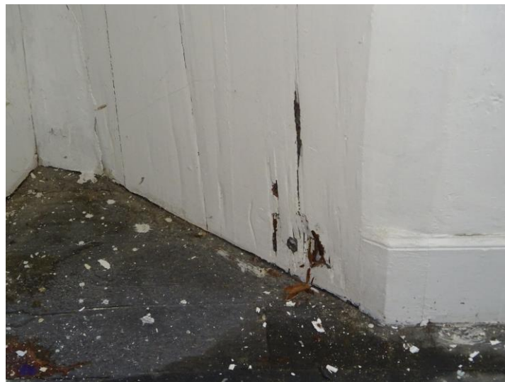
20. Rot to timber boarding onto Oates Travel building.
