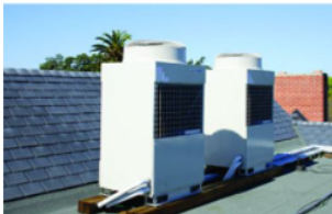
VRF zoning systems installed in 2004 at the University of Southern California.
