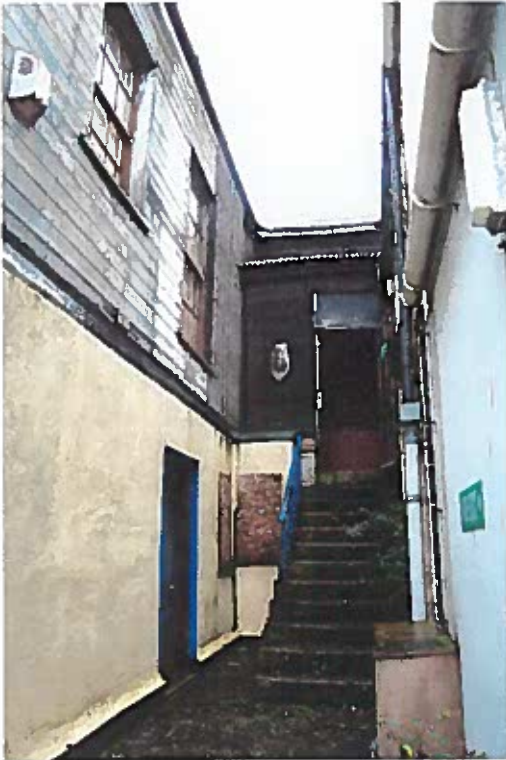
The internal foundry courtyard looking towards rear staircase. The former drawing office is on the left, the undercroft beneath the timber structure having been enclosed in the 1980s. The west wall of the offices to the right, with low eaves and dormer window probably dates from the earliest phase of the foundry.
