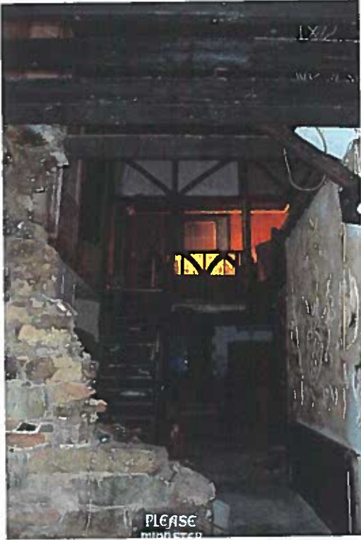
View from the main entrance into the rear of the former shop area . The first floor office with 'mediaeval' styling is visible through a large hole in the floor, formed as part of the Excalibur works, as was the partial demolition of the masonry in the foreground.
