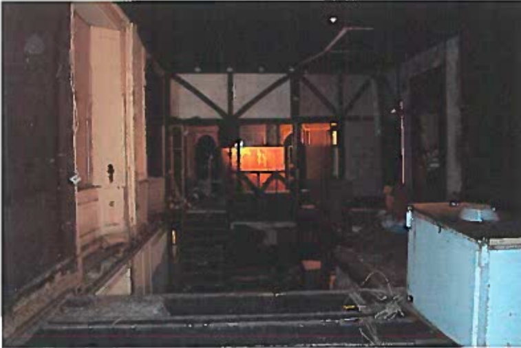
The main first floor office with 1980s 'adaptations' including the partial removal of the floor, insertion of staircase, 'mediaeval' styling and partial demolition of the partition to the former chairman's office beyond. The 19 th century windows and shutter boxes remain intact.
