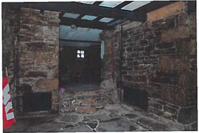
Remains of early foundry structures including probable furnace bases beneath the drawing office. The polished granite floor and the rubble wall in the background are insertions from the 1980s.
