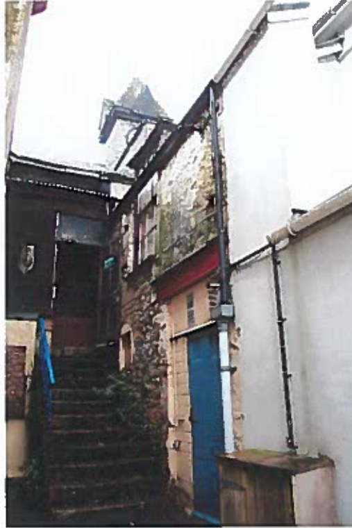
The internal foundry courtyard looking towards rear staircase. The former drawing office is on the left, the undercroft beneath the timber structure having been enclosed in the 1980s. The west wall of the offices to the right, with low eaves and dormer window probably dates from the earliest phase of the foundry.
