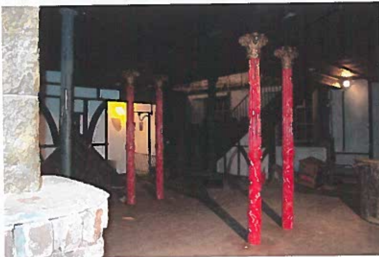
The former shop area. The ornamental cast iron columns, which support the main structural wall above are probably of a type used on waterworks pumping engines. The plain columns support a first floor strong room. The staircase and 'half timbering' are insertions from the Excalibur works.
