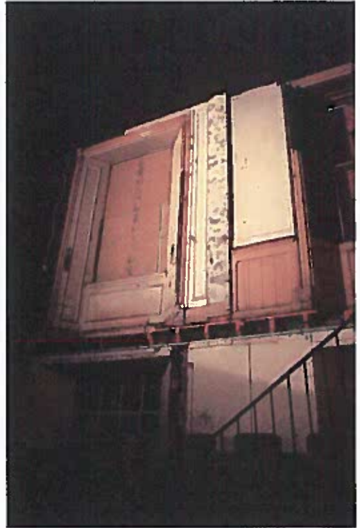
The main first floor office with 1980s 'adaptations' including the partial removal of the floor, insertion of staircase, 'mediaeval' styling and partial demolition of the partition to the former chairman's office beyond. The 19 th century windows and shutter boxes remain intact.
