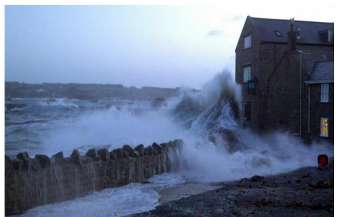
Overtopping of Mermaid Sea Wall, 2014 (photo courtesy of the Duchy of Cornwall)
