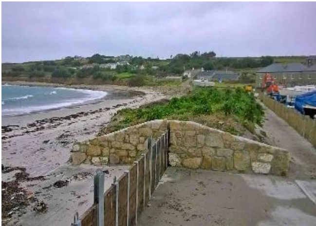
Demountable defence & south end of embankment
