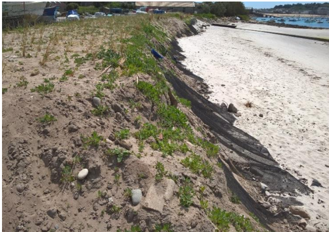
Exposure of geotextile matting after 2 years
