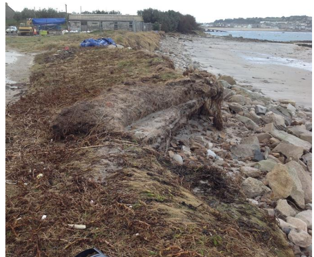
Damaged Porthloo bank after 2014 storm
