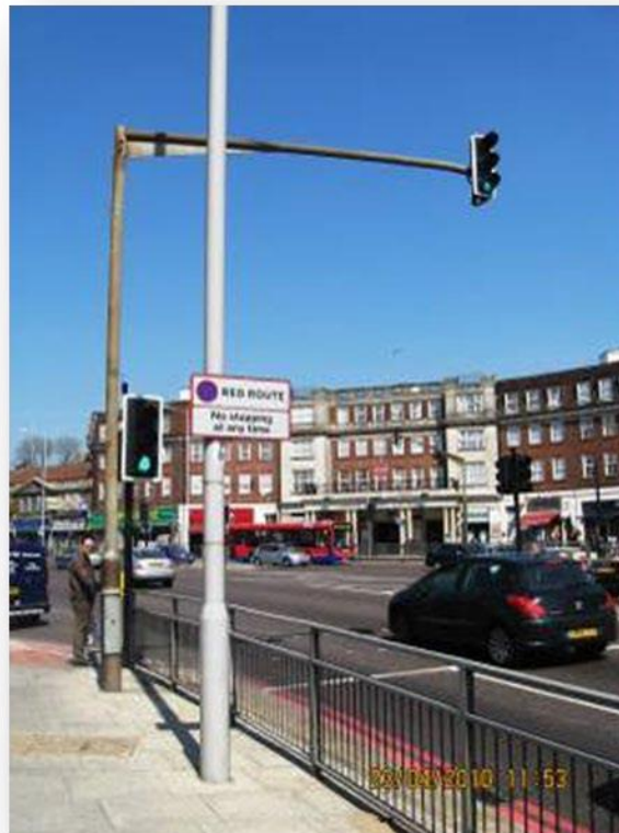
Post Type: Signal Mast Arm
