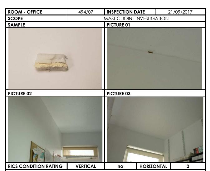
SAMPLE - Mastic joint not dry or cracked; flexibility and plasticity of sealant maintained. The movement joint width is 16mm, white foam filler (Compriband) was found, and in good condition.
