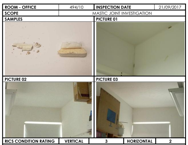
RIGHT SAMPLE – Horizontal mastic joint not dry or cracked; flexibility and plasticity of sealant maintained.
