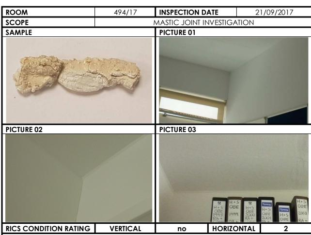
SAMPLE - Mastic joint not dry or cracked; flexibility and plasticity of sealant maintained. The movement joint width has been reduced (from expected 16mm), white foam filler (Compriband?) not found.
