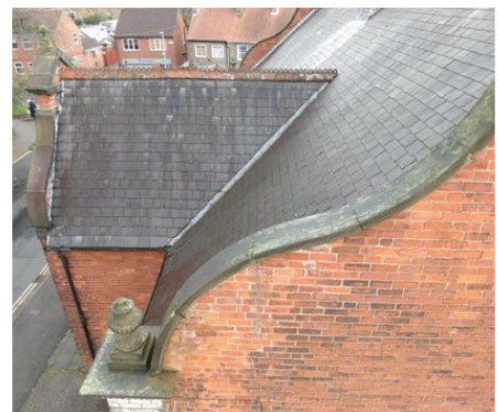
Gable parapet and entrance roof.
