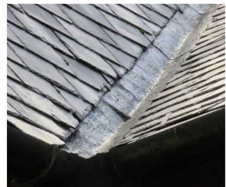
Liquid repair to valley gutter.
