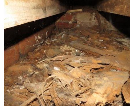
Debris and signs of wet rot to hall floor.
