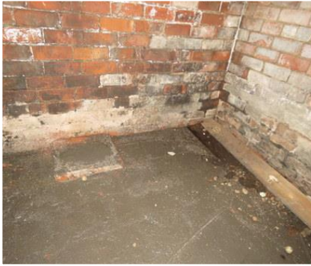
Potential floor detritus in reception room void.
