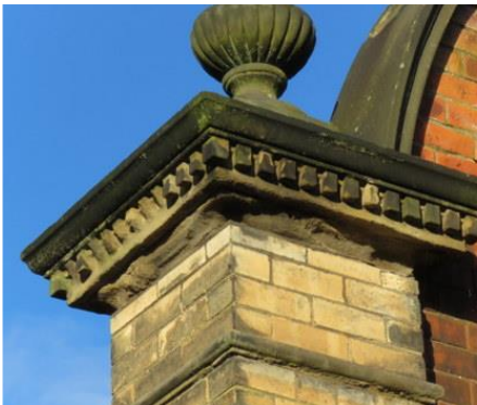
Eroding stone to most stone details.
