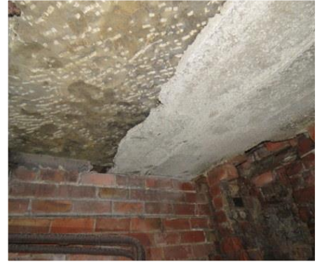
York stone and concrete fire place half beneath chimney.
