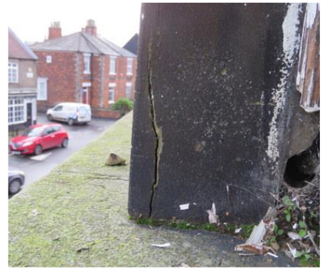
Cracking to face of stone column between Wilbert Lane gable window.
