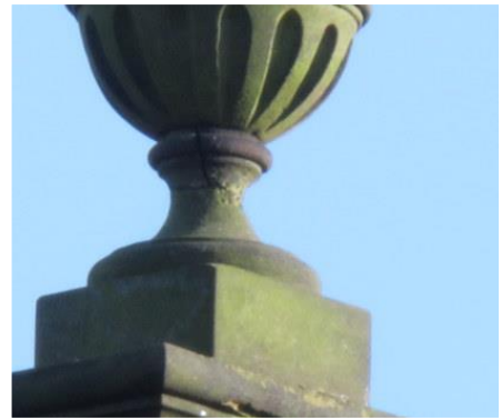
Cracking to stone support on finial on Wilbert lane gable.
