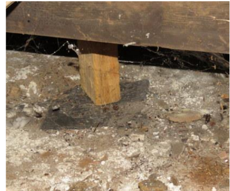
Additional supports fitted beneath damp joists to floor at Wilbert lane entrance.
