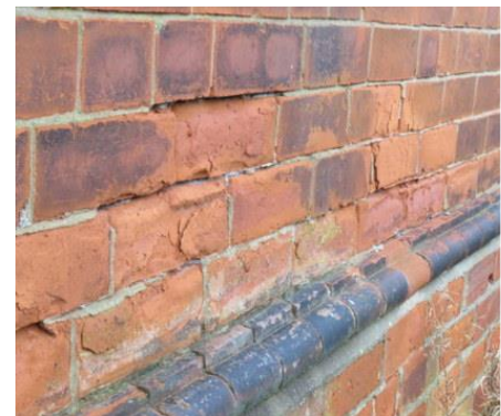
Poor pointing/spalled brick faces to a number of locations.
