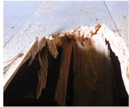
Beetle activity to floor void at corner of Wilbert and Morton lane.
