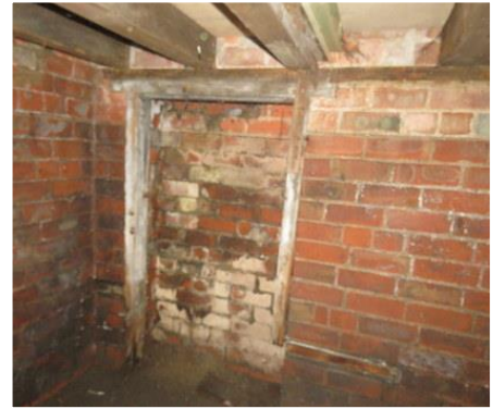
Old doorway beneath floor. Air brick evident within void.
