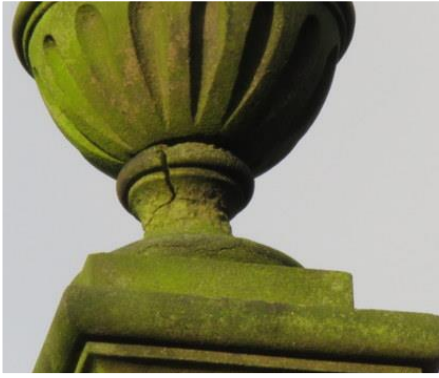
Cracking to stone support on finial on Wilbert lane gable.
