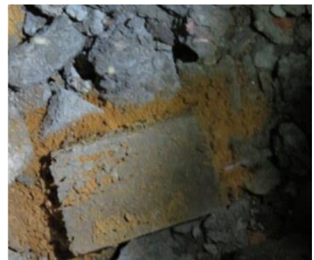
Beetle activity in floor void.
