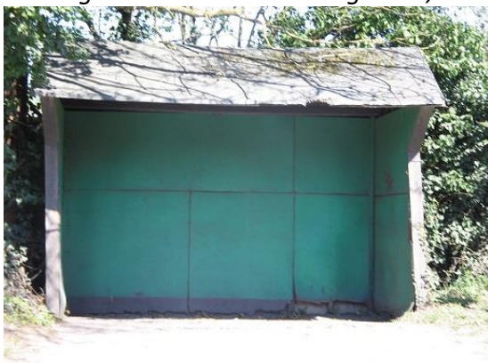
Existing bus shelter on Reading Road, South bound, opposite Walden Avenue
