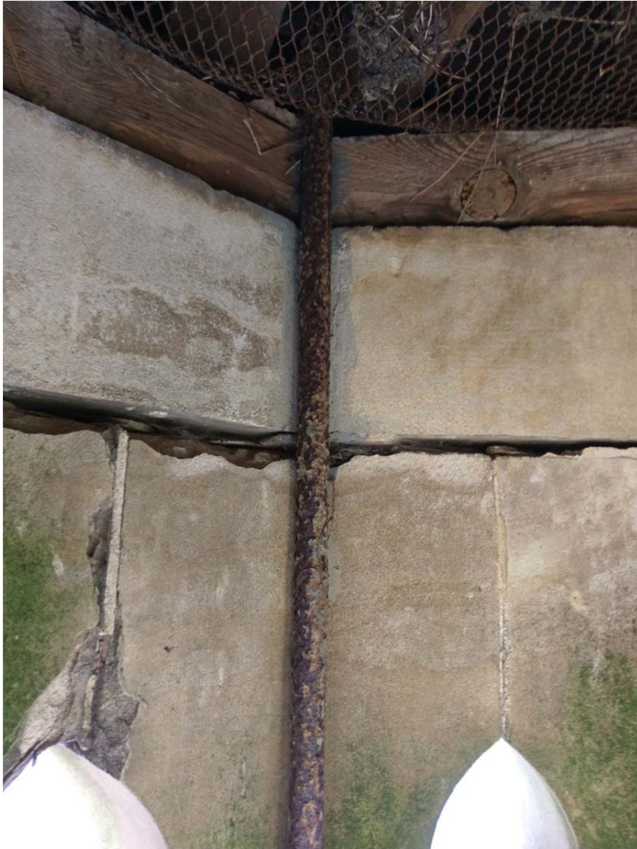
P7 – Horizontal bed joint cracking
