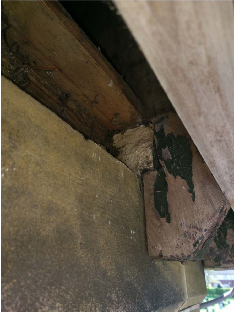
P6 – Loose corbel stone removed from southwest elevation
