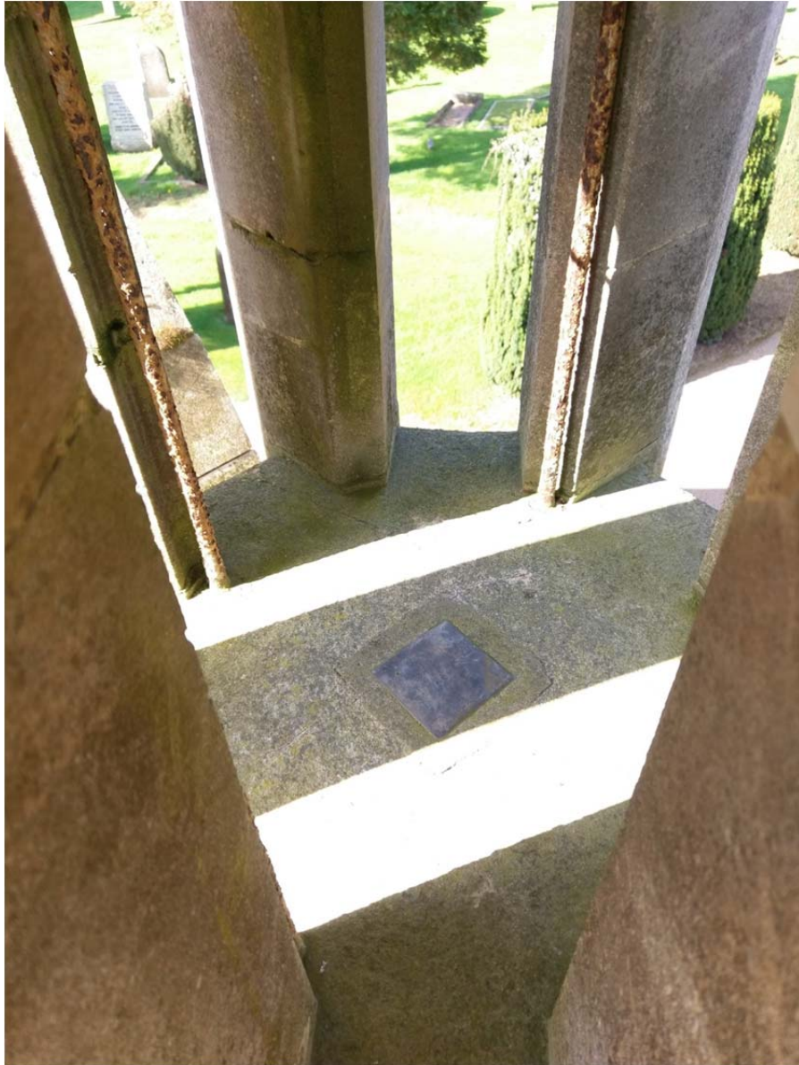
P2 – Plinth / cap stone with central tie bar
