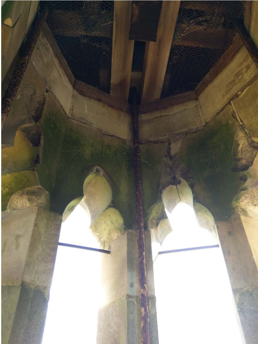
P8 – Eroded stonework internally
