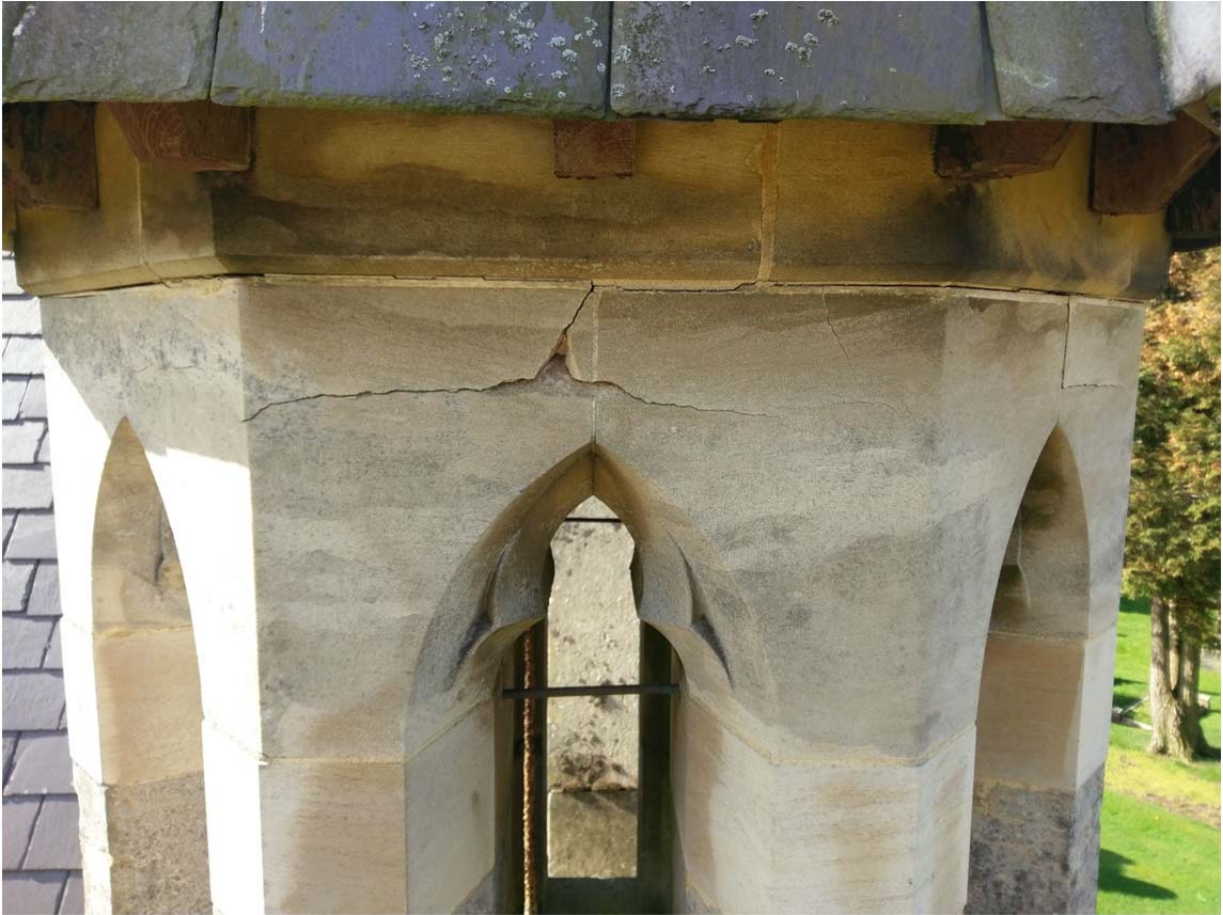
P5 – Horizontal cracked bed joint and spalling face (north elevation)
