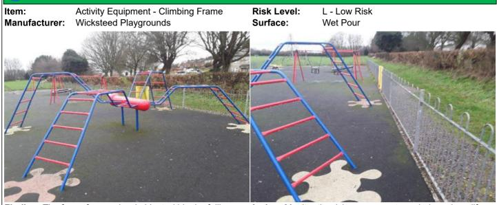
**Finding:** The fence forms a hard object within the falling **Action:** Monitor the rispace of the equipment in contravention of the requirements the design if required of BS EN 1176 Part 1
