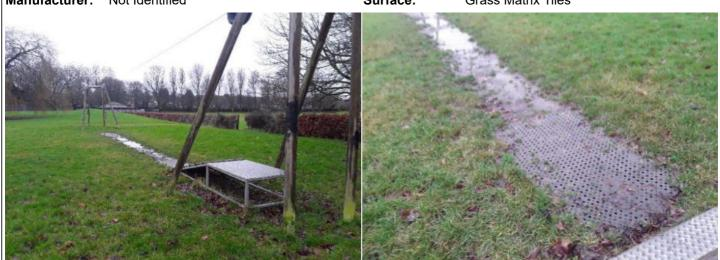
Finding: A grass matrix tile has been installed upside down Action: Re install the grass matrix tile the correct way up
