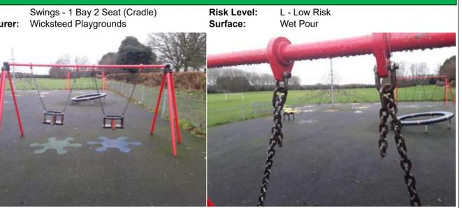
Finding: There are excessive chain tails provided, however Action: Cut back excess chain tails but ensure a minimum a minimum of 2 additional links should always be provided of 2 additional links remain through the crucifix with crucifix connectors
