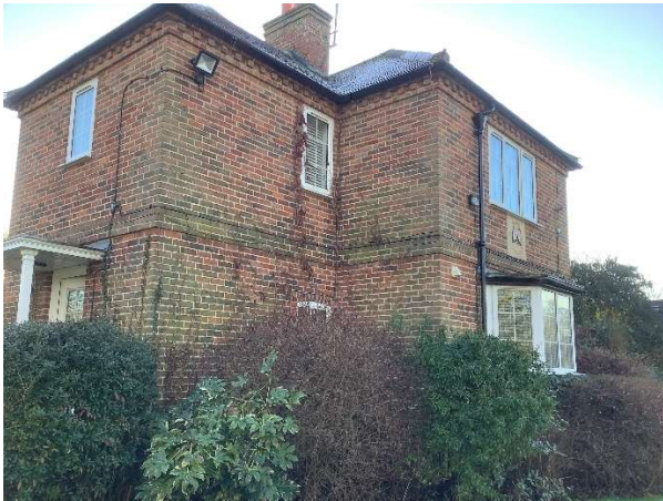
Front elevation overlooking lock
