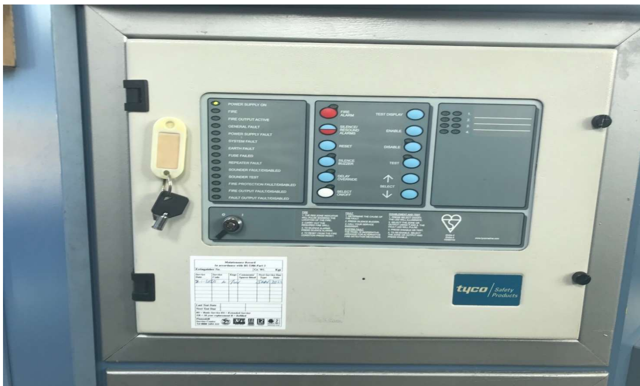
New Fire Detection Monitoring Control Panel
