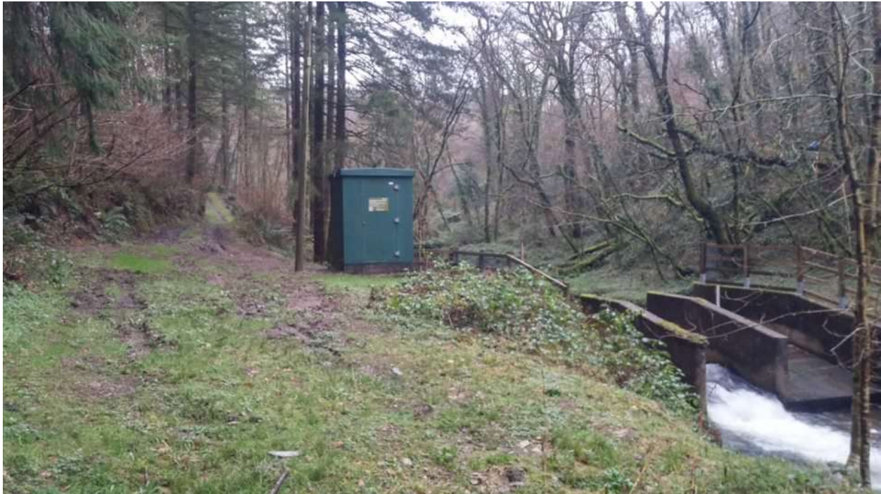
Photo 13: Extent of lay down area which slopes slightly.
