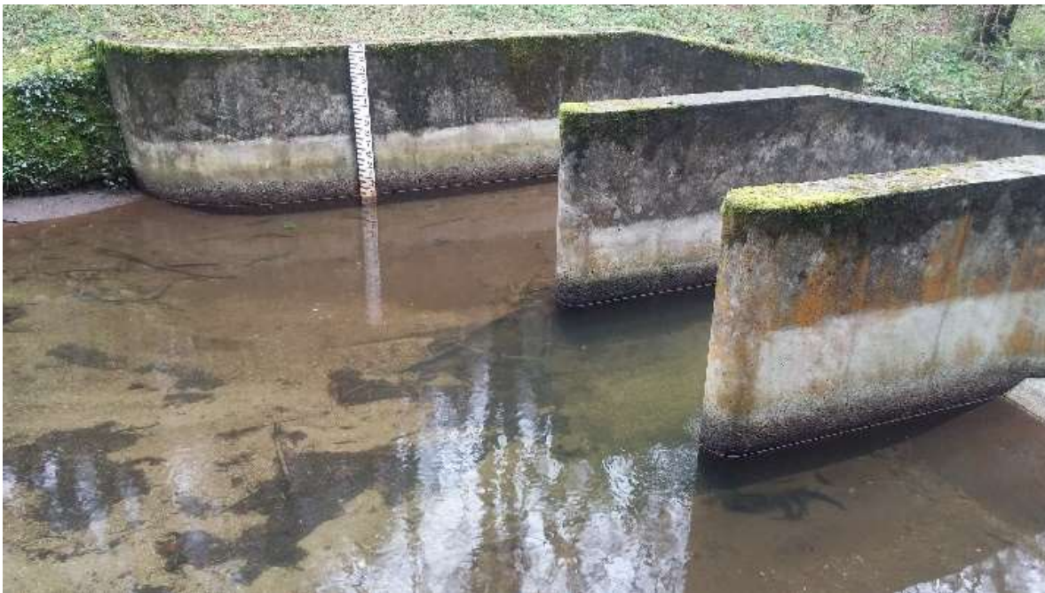
Picture 6: View of gauging section upstream of structure in low flows.
