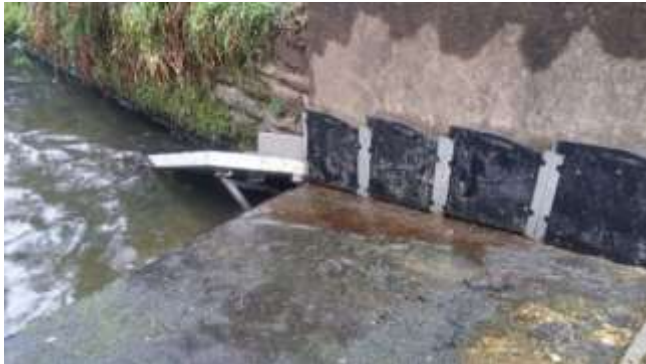
Picture 7a and 7b: Eel cassette pass attached to right hand side wingwall of Craigshill Wood gauging station.
