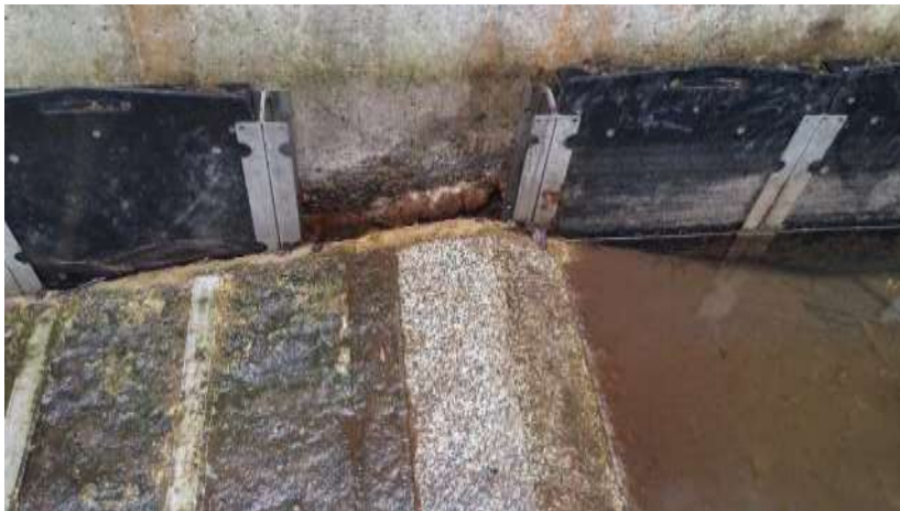
Picture 8a and 8b: Removed eel cassette to show internal tile and bristle formation
