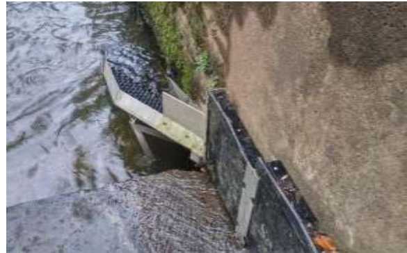
Picture 7a and 7b: Eel cassette pass attached to right hand side wingwall of Craigshill Wood gauging station.
