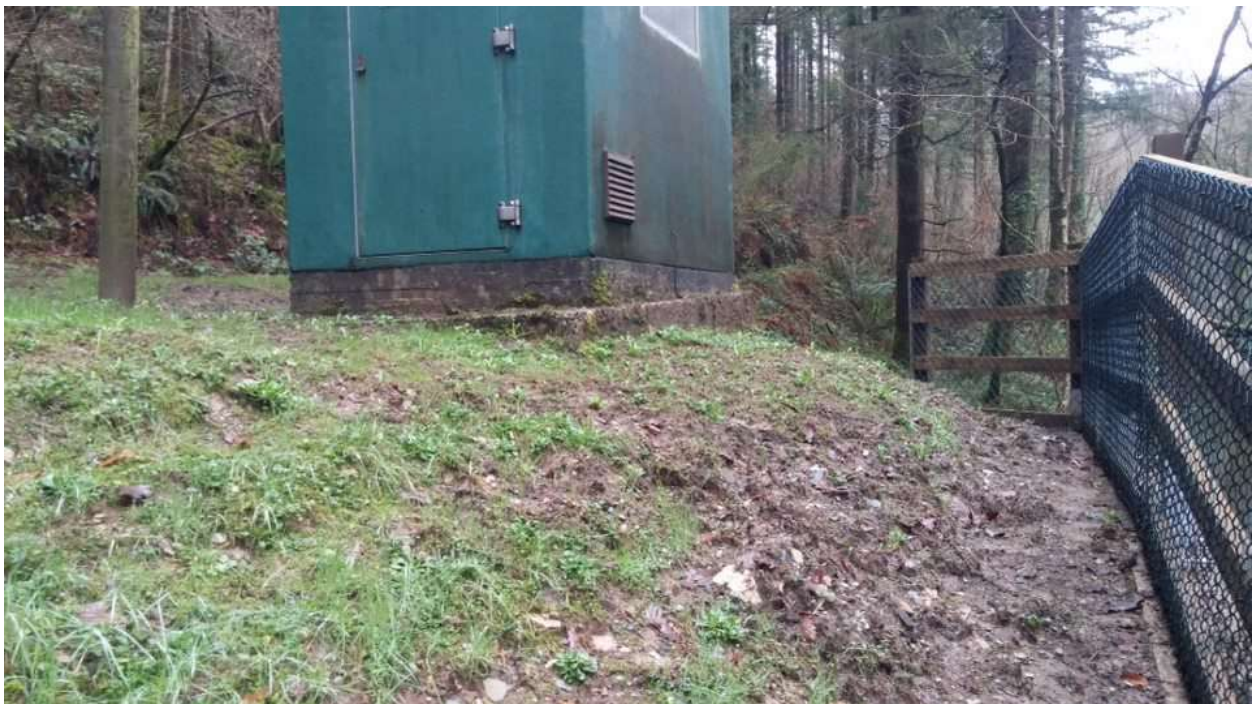
Photo 14: Drop off of lay down area next to gauging hut.
