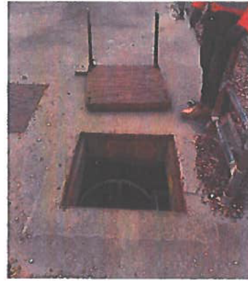
Photo 24 – Bulverhythe – Outer Chamber. Existing top hatch access.
