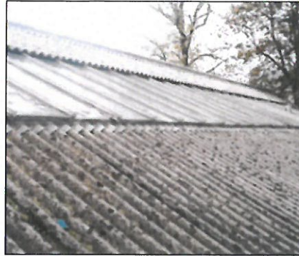
AC sheets used as roofing
