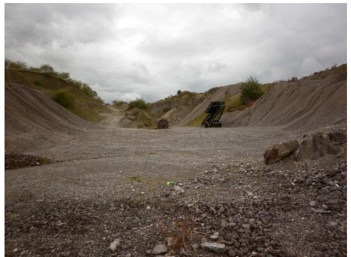
Gap to be infilled using material available on site (above: view from west, right: view from east)
