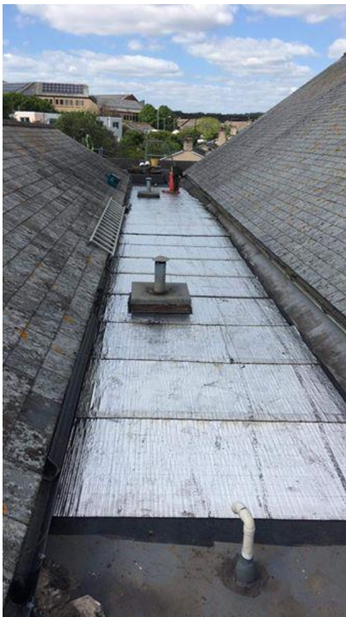
Barham -This was a warm roof system comprising of @danosauk vapour layer, 120mm insulation, Danosa underlay and then Danosa mineral cap sheet.
