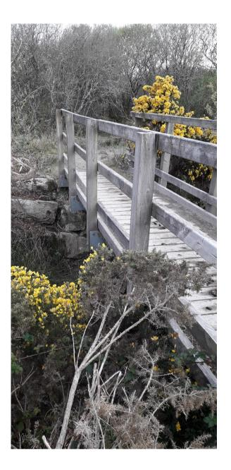
3.4.5 The handrails were loose. The nuts on most of the fixing bolts were not tight.
