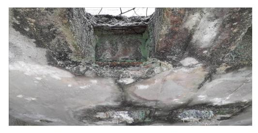
3.12.16 Many steelwork elements were noted embedded in the walls. The corrosion of theses members will cause damage to the walls as the rust products expand. Where possible steelwork embedded into the walls should be removed and the walls made good.
