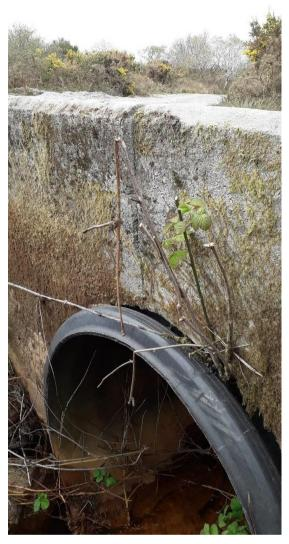
3.3.8 Slight cracking was noted on the North Headwall. This should be repaired.
