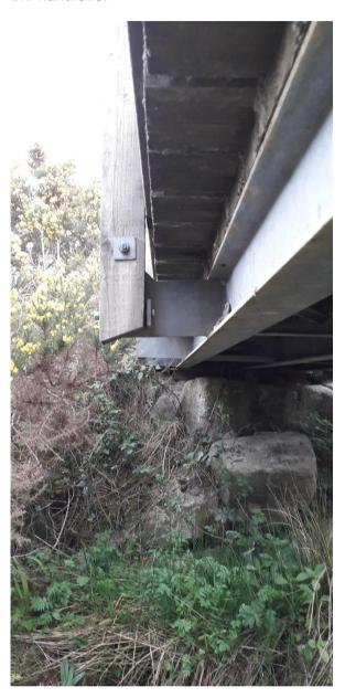
3.4.7 The handrail was twisted and screw fixings were rusty, with only one screw per fixing. Rusty screws should be replaced with stainless steel suitable for external exposure, and provide a minimum of two screws per fixing.
