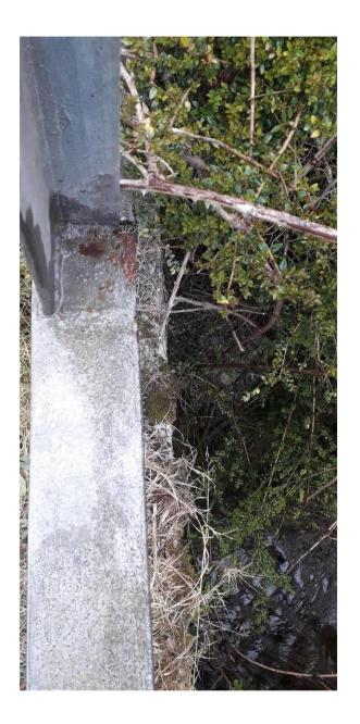
3.1.10 The Northwest baluster was loose. The fixings should be tightened or replaced.
