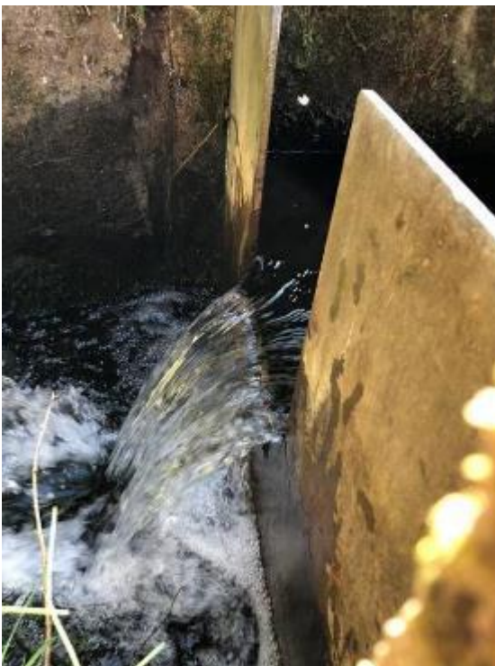
Figure 9 Existing weir showing aerated nappe
