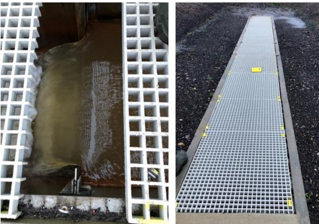
Figure 25 Thin Plate weir installation (weir on left and chamber on right)
