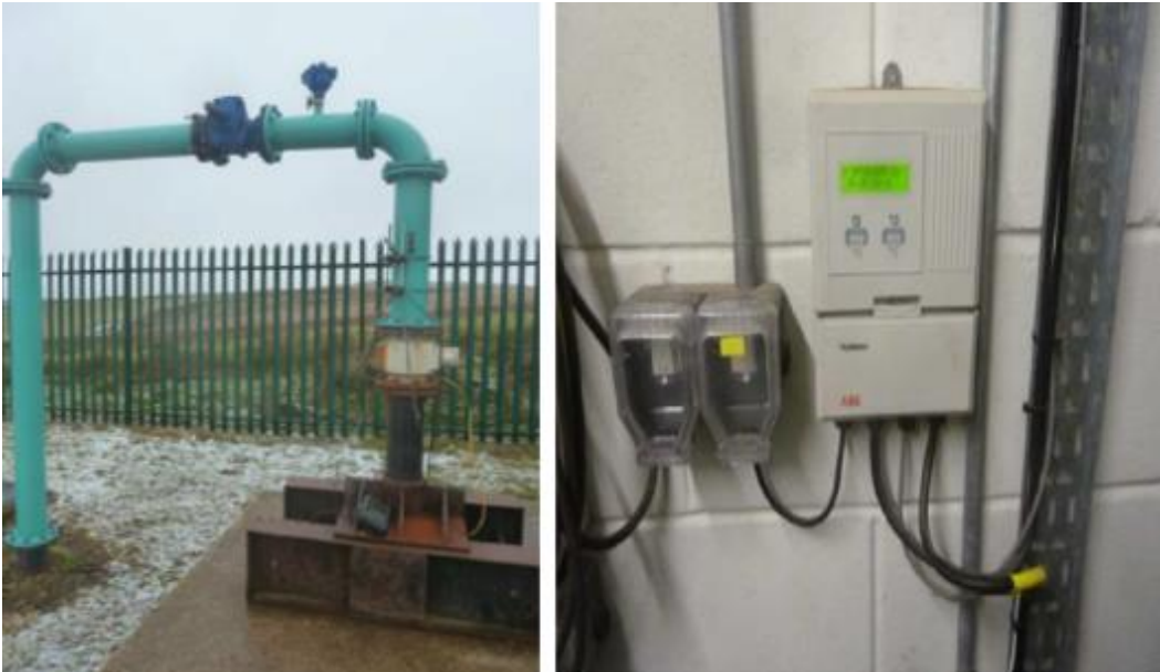
Figure 24 Pipeflow meter 2 - Meter installation (left) and transmitter (right)
