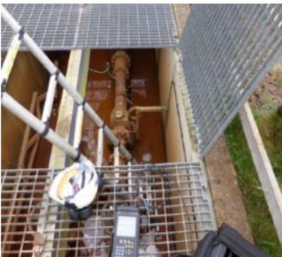
Figure 23 Pipeflow meter 1 – Meter installation (left) and transmitter (right)
