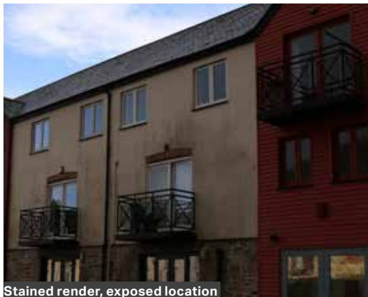
Stained render, exposed location
