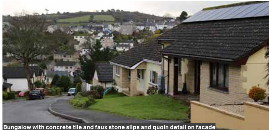
Bungalow with concrete tile and faux stone slips and quoin detail on facade
