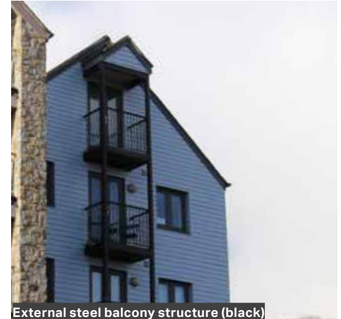
External steel balcony structure (black)
