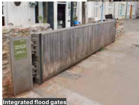
Integrated flood gates
