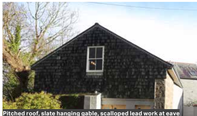
Pitched roof, slate hanging gable, scalloped lead work at eave
