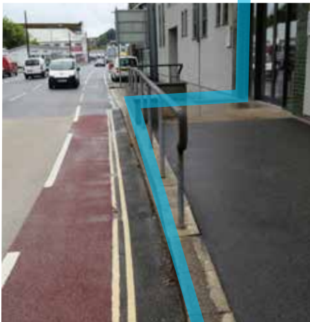
Example of raised access with better flood resilience
