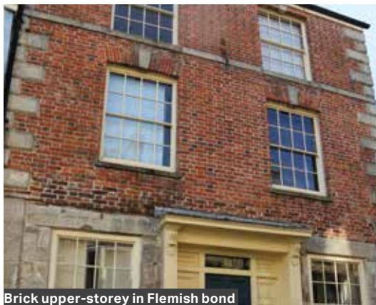
Brick upper-storey in Flemish bond
