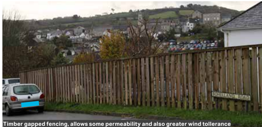
Timber gapped fencing, allows some permeability and also greater wind tolerance
