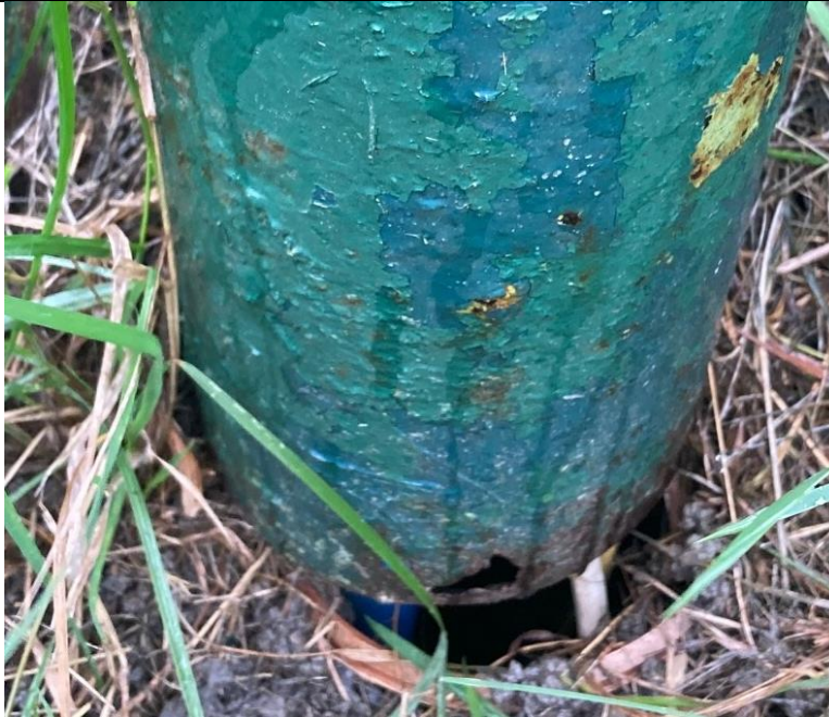
Figure 3: Exposed cables at the base of stilling well tube
