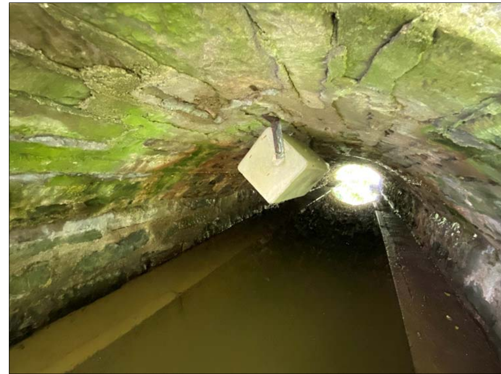
Photograph 2 - Bird box attached to arch barrel - 600mm from downstream elevation (note slight mortar loss and repair)
