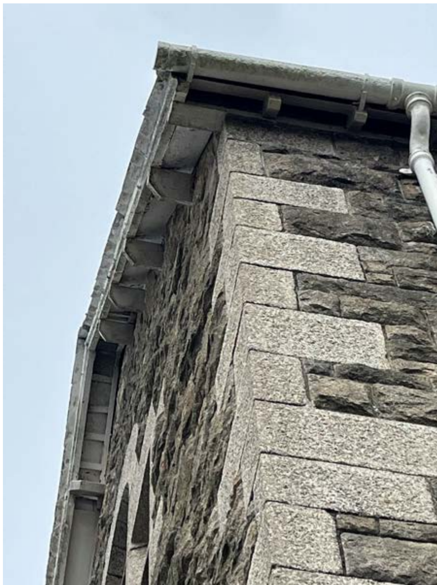
Basset House eaves with board finish, detail to be confirmed when intrusive survey can be carried out.
