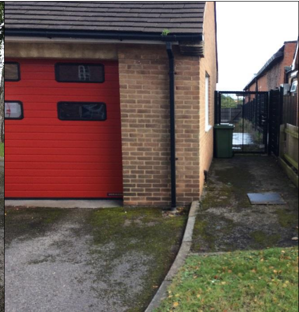
B – View of Side Elevation Footpath
