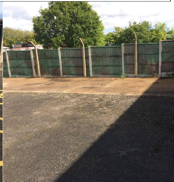
D- View of Rear Yard
