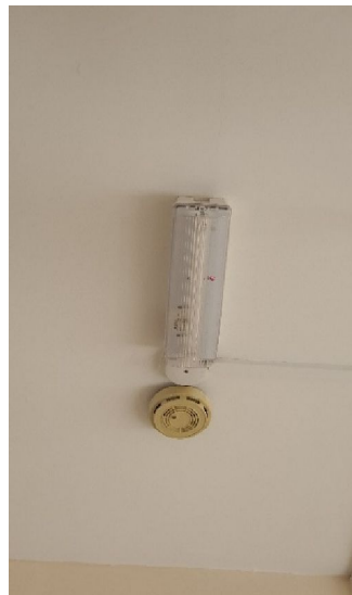
Emergency lighting and old detector
