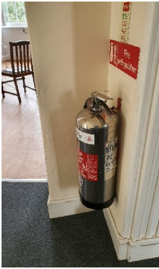
Fire extinguisher to replaced or serviced
