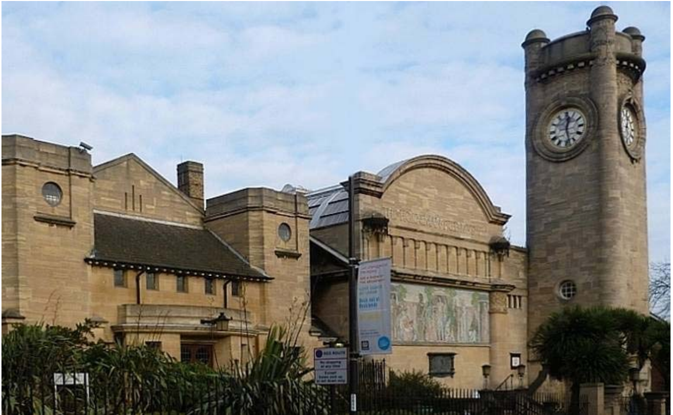
Fig 01 – View from 100 London Road
