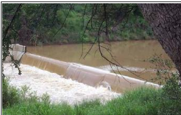
Sharp crested weir [SHARP]
