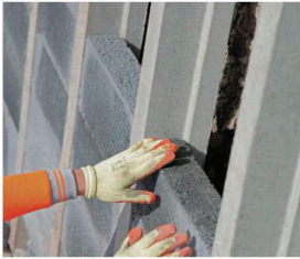
Figure 9 – Photo of beam and block floor (source: Forterra.co.uk)
