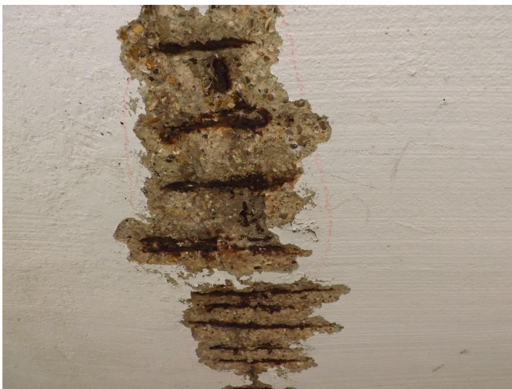
Photograph 4 – Typical instance of corroded reinforcement in deck soffit.
