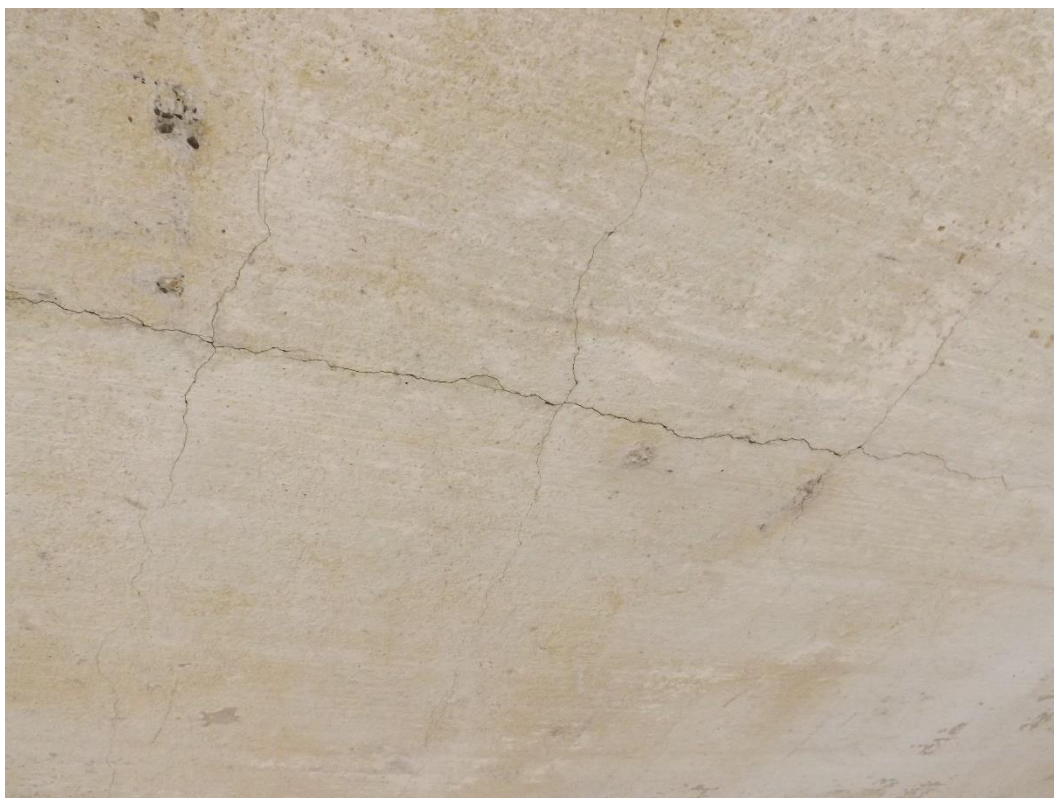
Photograph 7 – Typical instance of cracked deck soffit.
