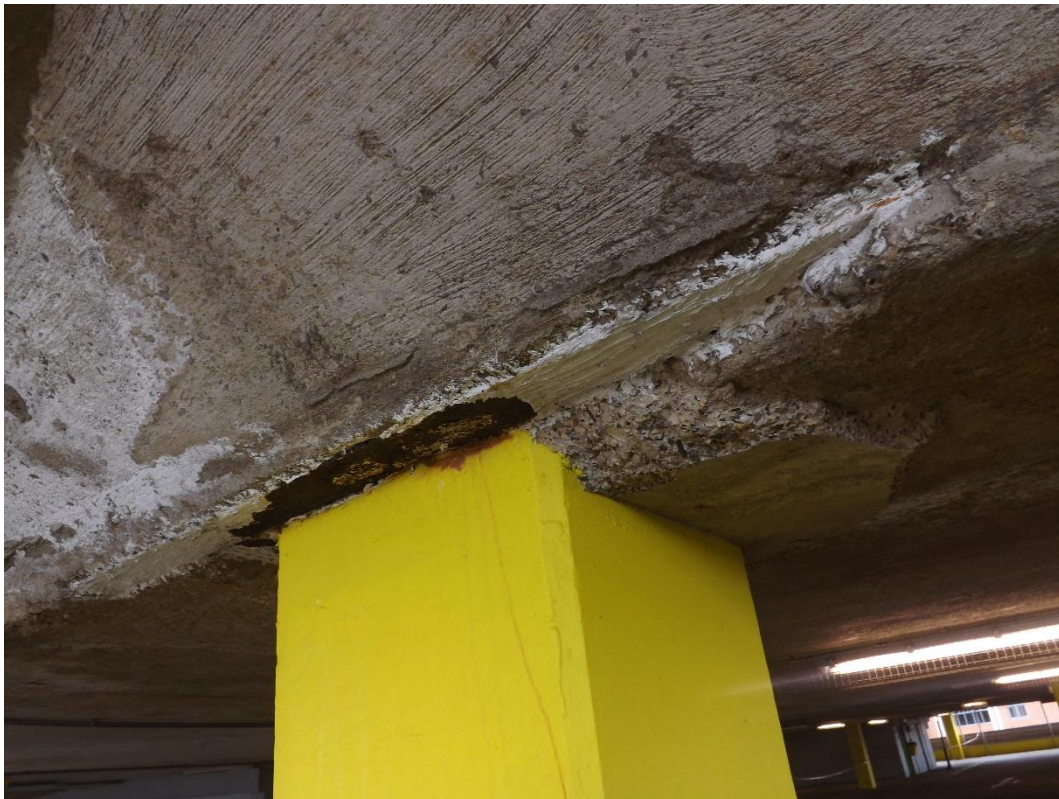
Photograph 19 – Exposed and corroded column head deck support frame.
