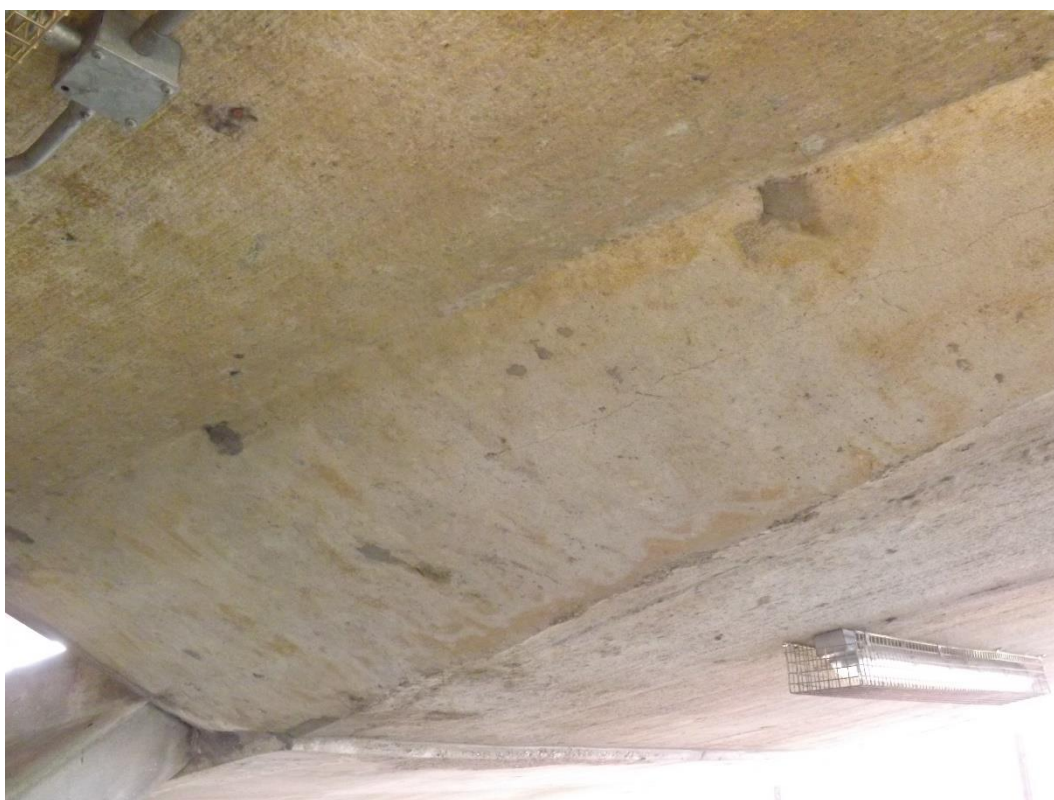
Photograph 14 - Longitudinal crack along ramp edge.
