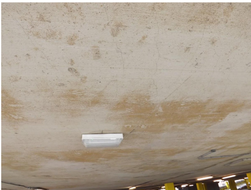
Photograph 8 - Typical instance of cracked deck soffit.
