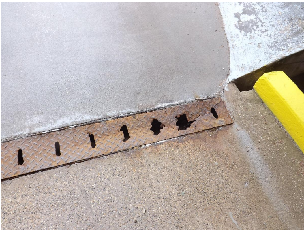
Photograph 21 – Example of defective corroded drainage items.
