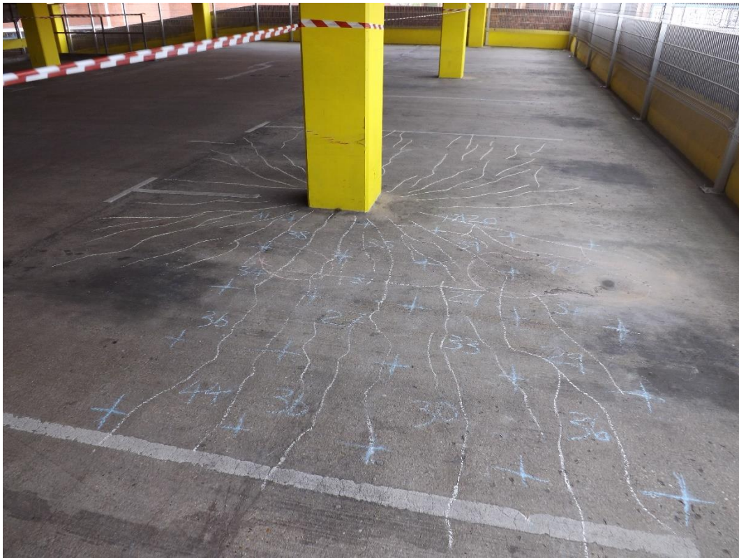
Photograph 15 – Typical deck cracking at column locations.
