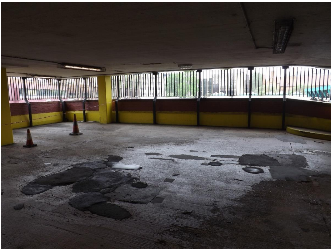
Photograph 12 - Typical historic 'patch' repairs in deck.
