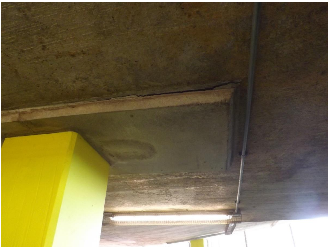
Photograph 18 – Cracked/part detached soffit down-stand at column head prior to removal.
