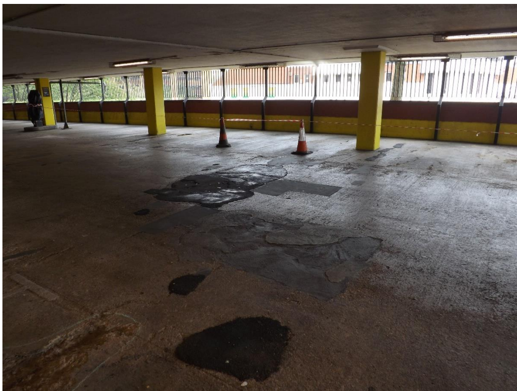
Photograph 13 – Typical historic 'patch' repairs in deck.
