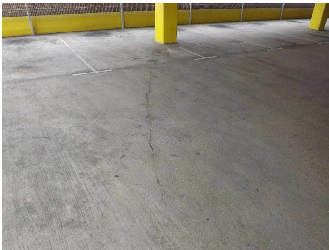
Photograph 10 – Typical cracking within deck.
