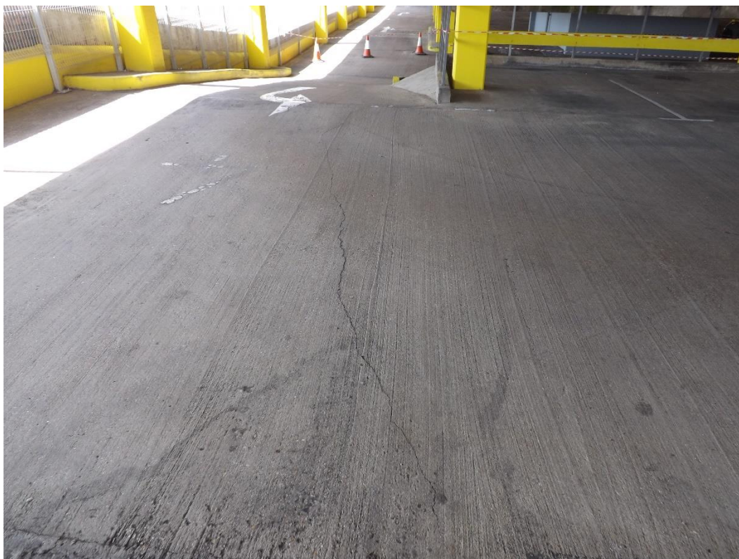
Photograph 9 – Typical cracking within deck.
