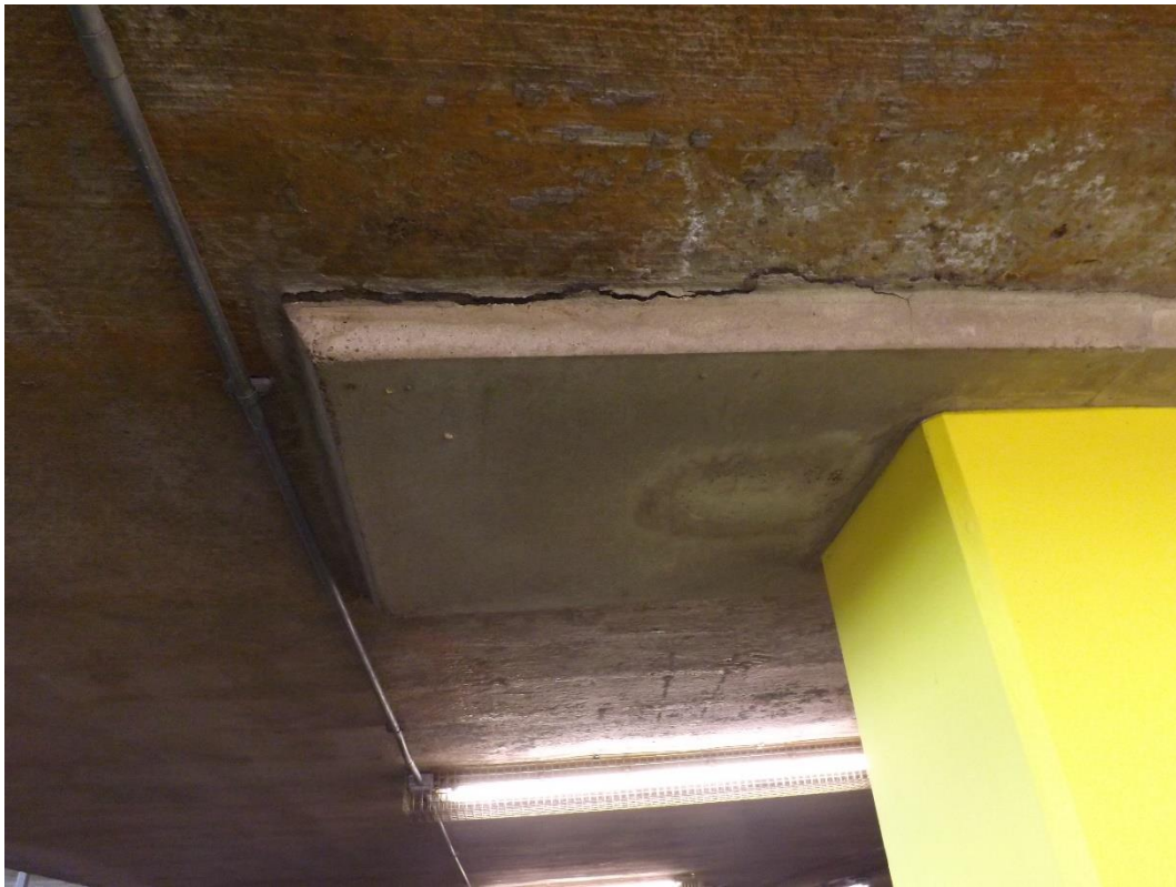
Photograph 17 – Cracked/part detached soffit down-stand at column head prior to removal.
