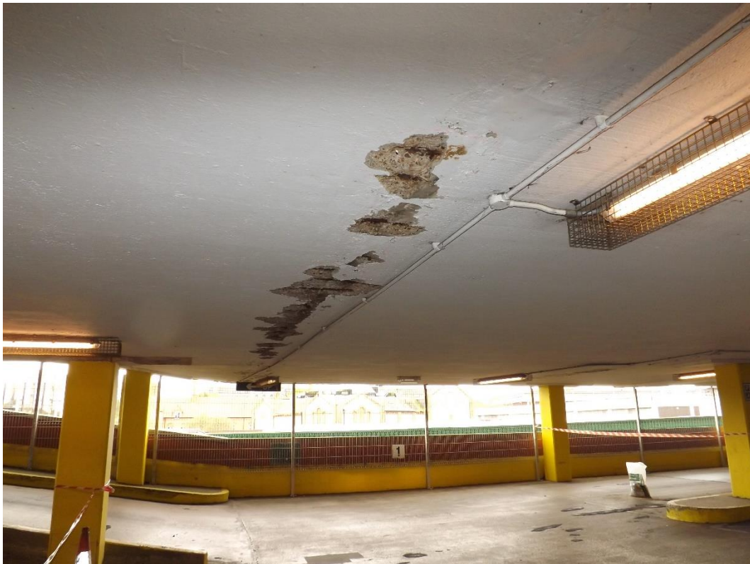
Photograph 5 - Typical instance of corroded reinforcement in deck soffit.
