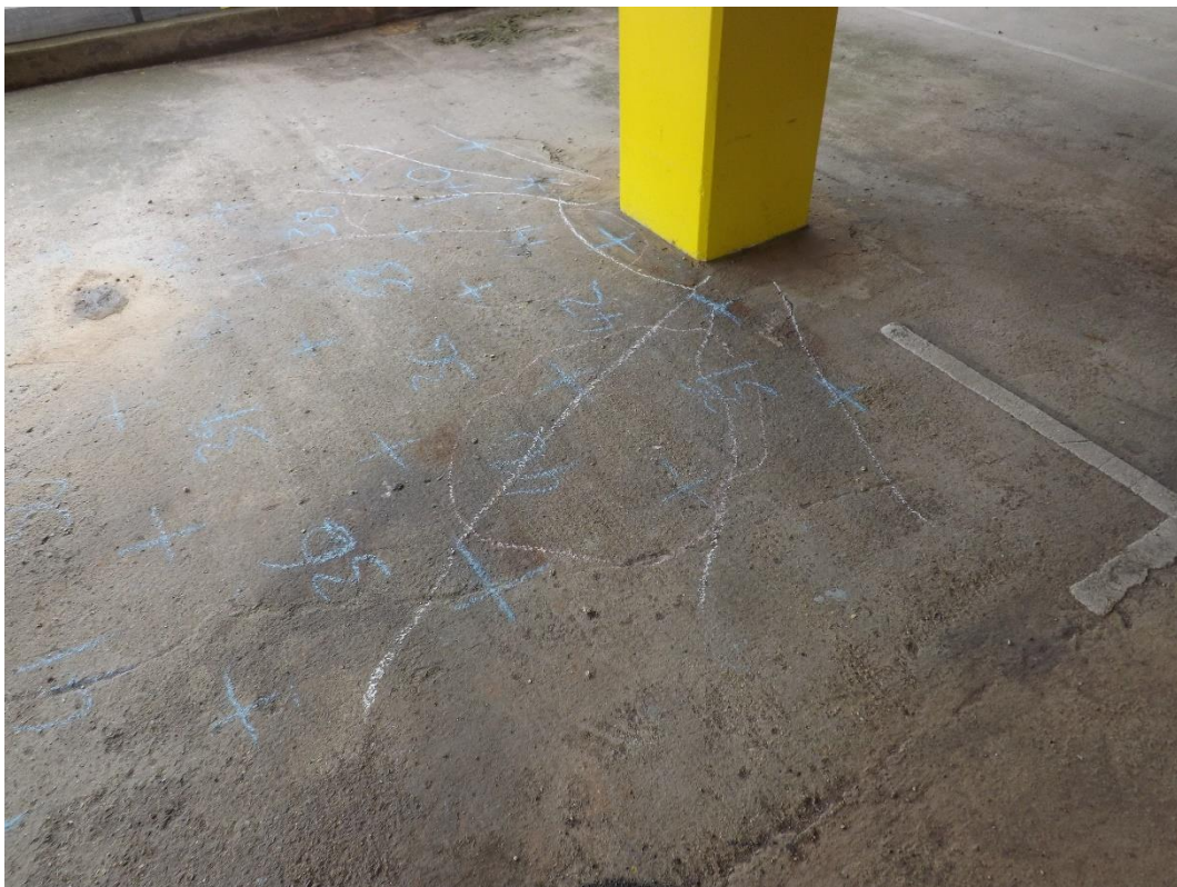
Photograph 16 – Typical deck cracking at column locations.
