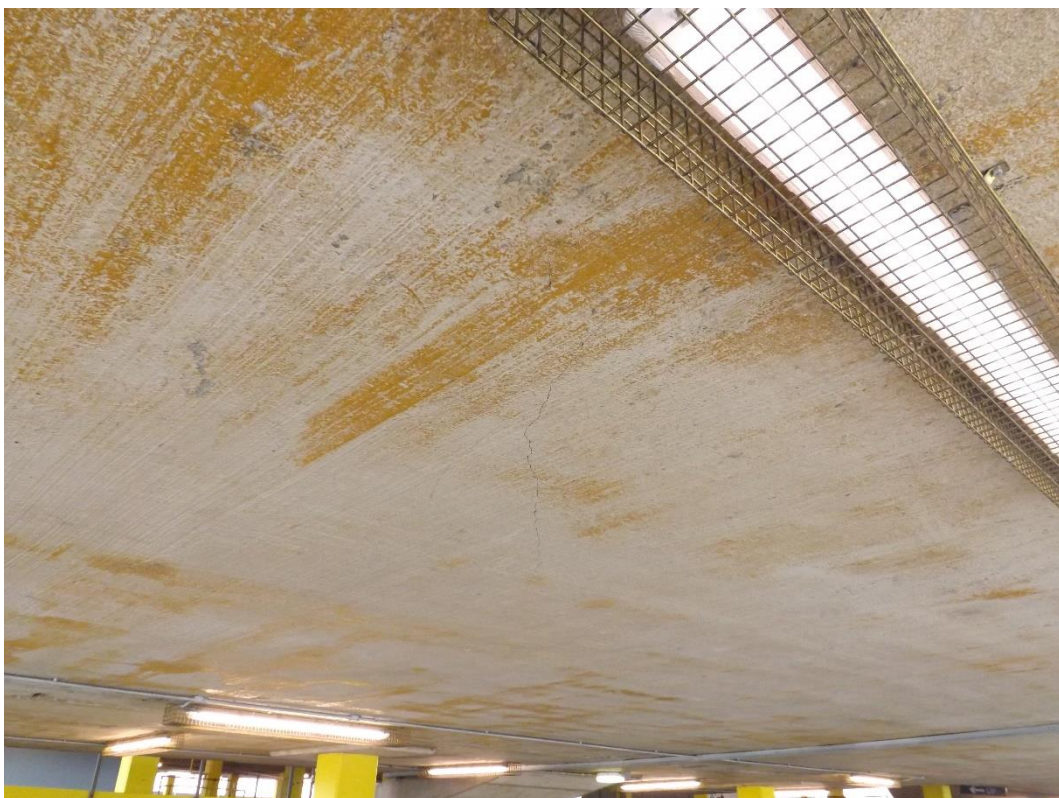
Photograph 6 – Typical instance of cracked deck soffit.
