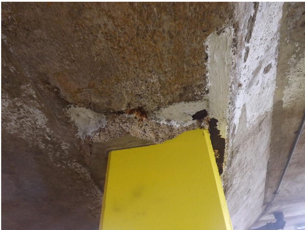
Photograph 20 – Exposed and corroded column head deck support frame.
