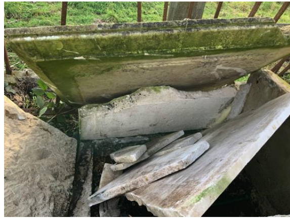
Detail of fractured south base panel of monument
