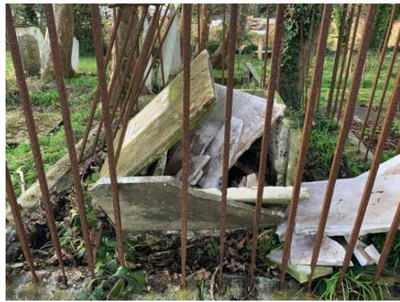
Detail of fragmented marble panels within and outside monument base
