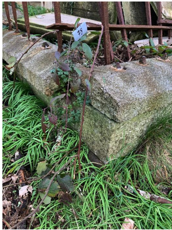
Spalled section of granite plinth, south west corner
