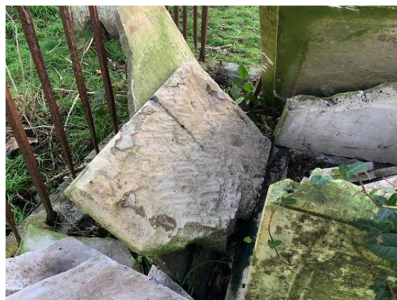
Detail of fractured east base panel of monument
