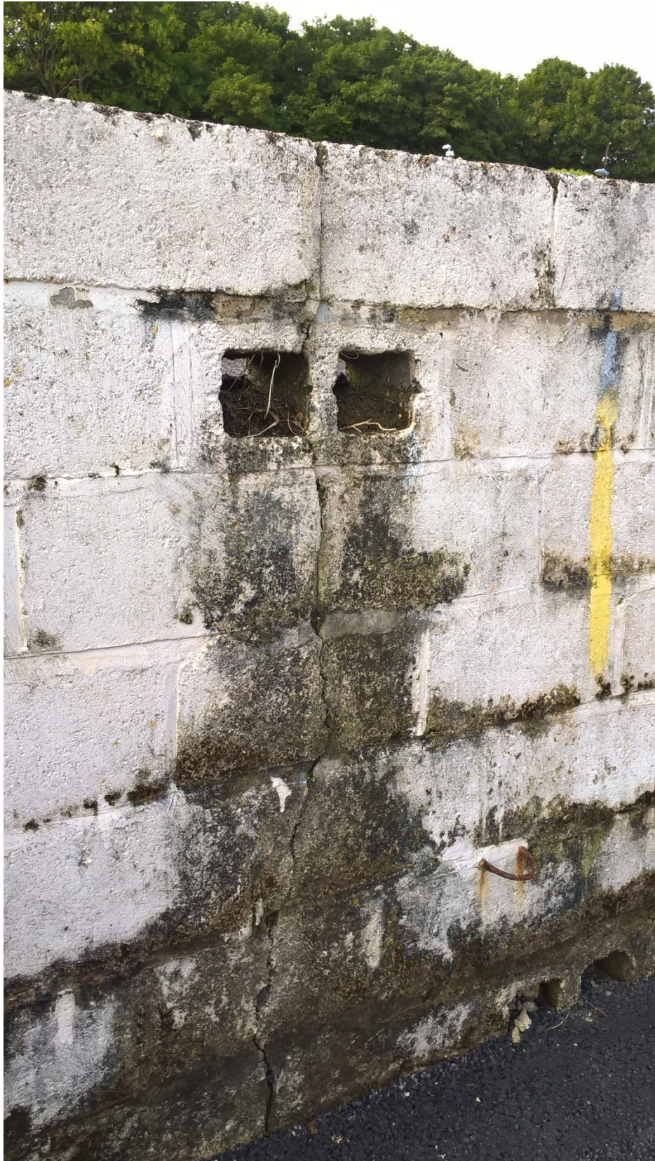
Wall crack
