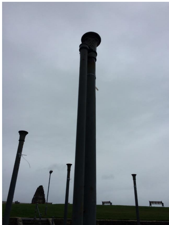
Image shows downpipe for drainage fixed to column B. The fixings for the drainage (also pictured below) are not original.
