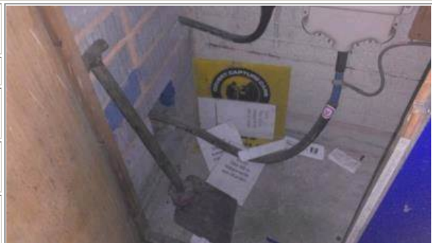
Photo No. 8 - Wrap to electrical cable - unable to sample for health and safety reasons
