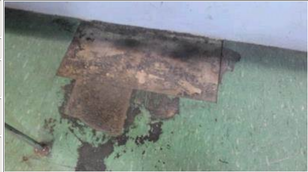
Photo No. 10 - Bitumen adhesive to floor, continuing below modern floor tiles (as sample HJ005235)
