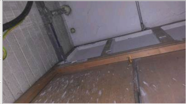
Photo No. 10 - Bitumen adhesive to floor, continuing below modern floor tiles (as sample HJ005235)
