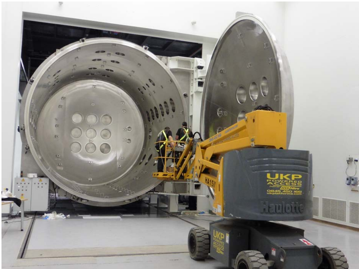
Figure 3: STC-3 vacuum chamber during installation
