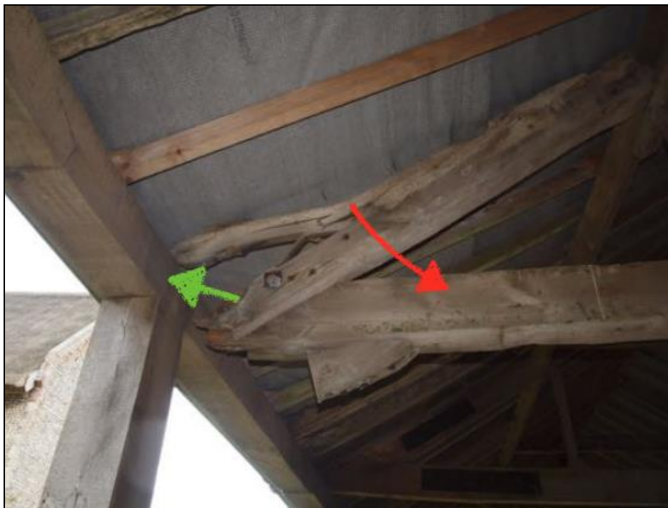
Figure 4: The roof truss has disconnected with the wall-plate and the roof has partially collapsed. Red arrow: Movement of the truss downwards. Green arrow: Movement of the wall-plate outwards (Photo: Nicholas Warns Architects).
