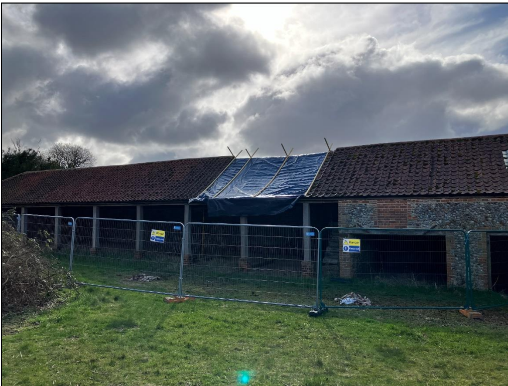
Figure 6: Temporary stabilisation and roof covering, and exclusion of public footpath from the South Range Barn (Photo: Natural England/ Howard Jones).
