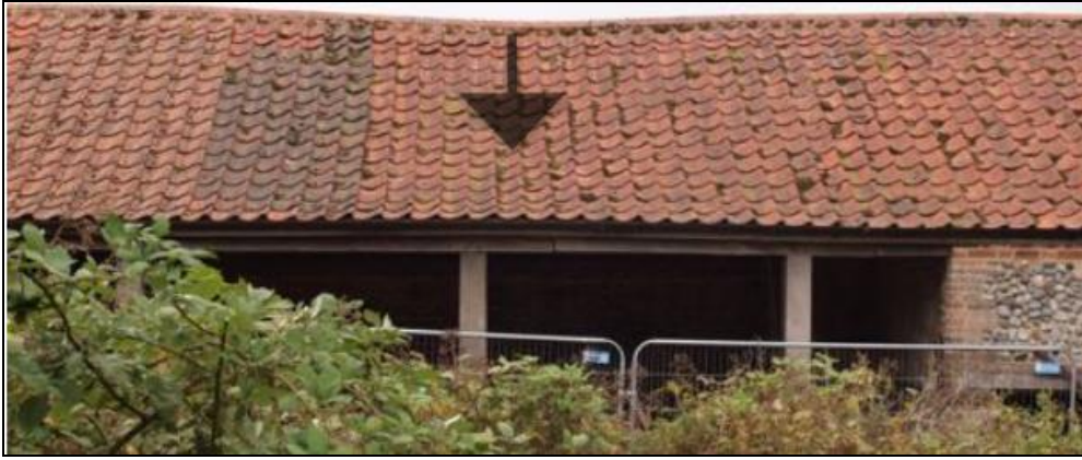
Figure 3: South Range Barn, showing collapsing roof (Photo: Nicholas Warns Architects).
