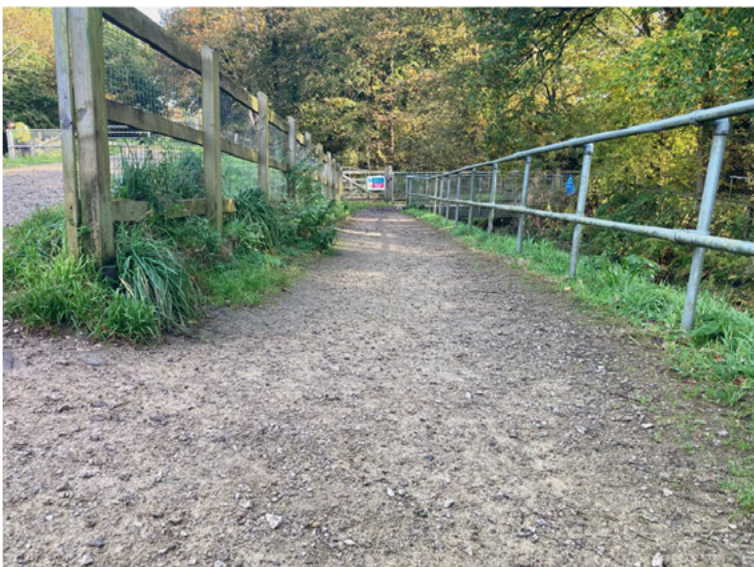
Image 6. Asset 134194, pedestrian ramp to be replaced with bound surface. Timber fence to be replaced and crest-shoulder transition remedied. Please use EA Access for all for specification guidance.
