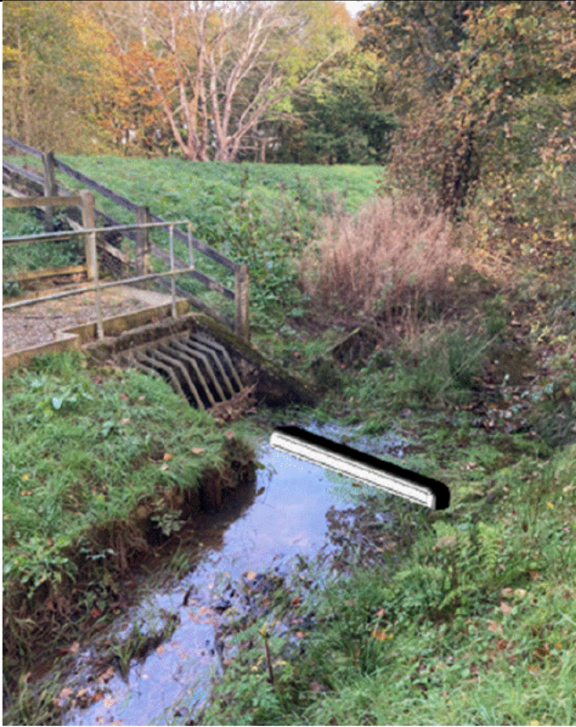
Image 6. Asset 134194, pedestrian ramp to be replaced with bound surface. Timber fence to be replaced and crest-shoulder transition remedied. Please use EA Access for all for specification guidance.
