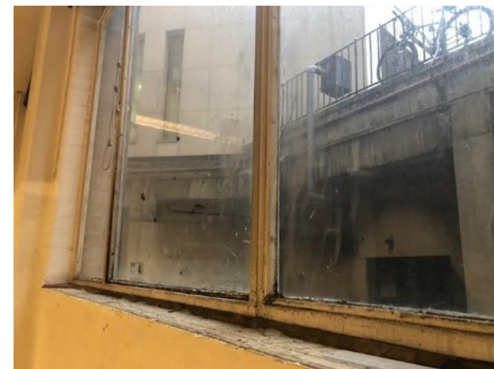
Window Photo - a single glazed, 1950's metal framed window
