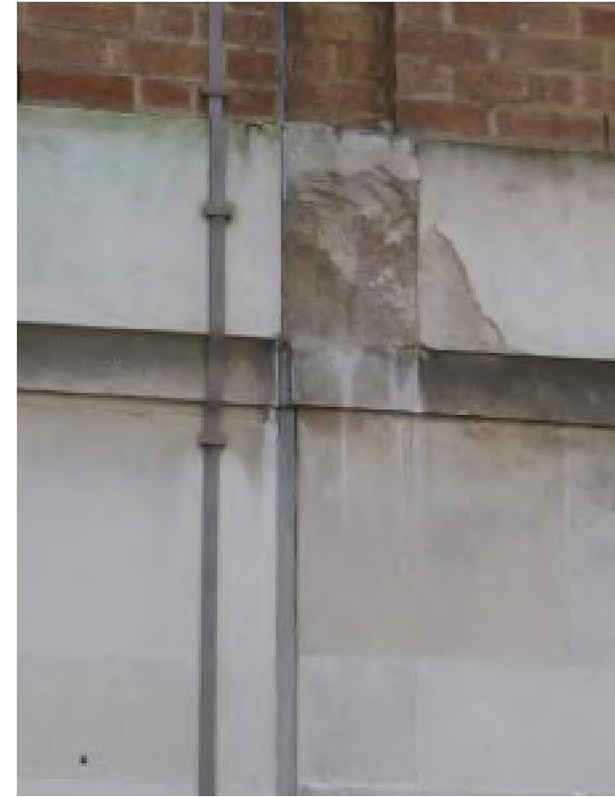
Exterior Photo - an example of an area of exterior stonework that has broken and fallen off
