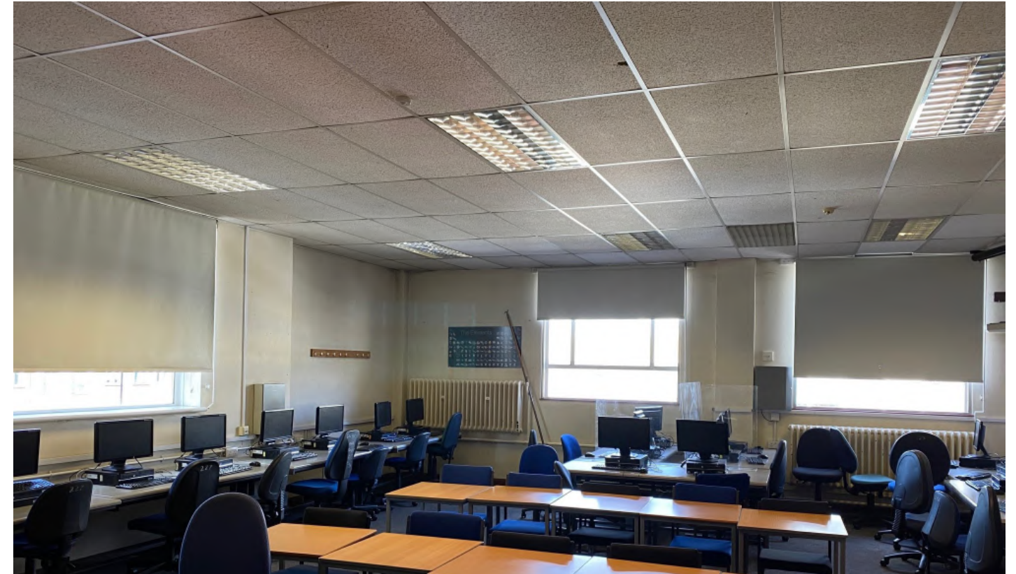
Classroom Photo 1 - 2nd floor classroom with single glazed, 1950's metal framed windows
