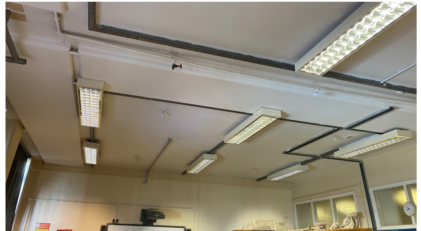
Classroom Photo 2 - 2nd floor classroom with exposed soffit - lacking a fitted ceiling - and surface mounted services and poor lighting provides a unwelcoming, poor and uninspiring learning environment
