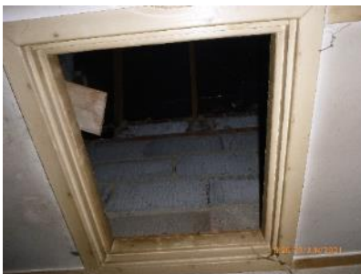
Figure 15. Roof void above toilet on ground floor, showing roof structure above.
