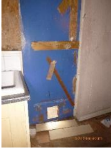
Figure 17. Boarded up door leading out through inverted dormer from kitchen of the living.
