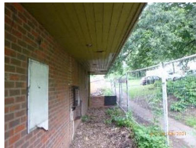
Figure 20. Example of overhanging eaves.
