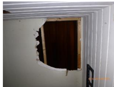
Figure 14. Example of damage to ceilings (lounge, ground floor).
