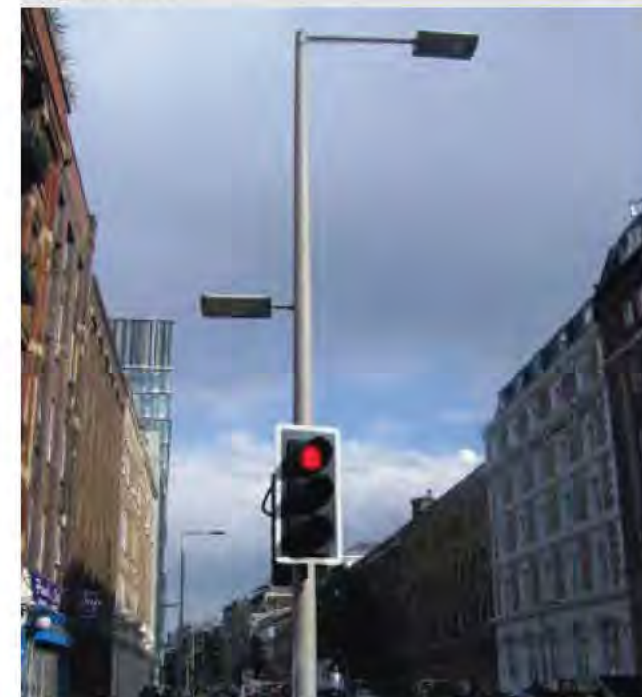
Figure 290: Combined lighting column and signal head
