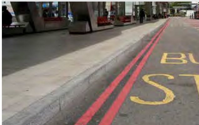
Figure 301: Bus interchange with a 140mm kerb upstand
