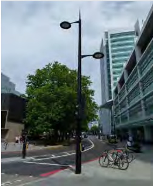
Figure 282: Highway lighting column illuminating footway and carriageway
