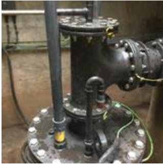
Greenlane borehole headworks
