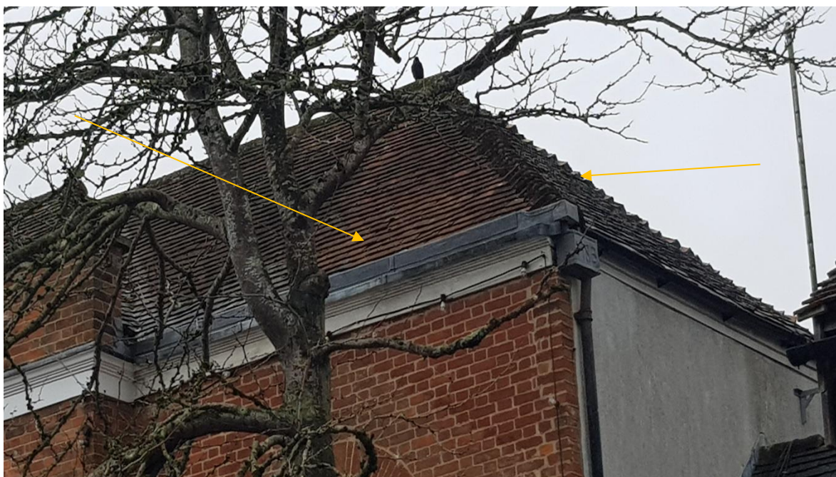
Picture 3: The a close-up of the northern elevation showing gaps under tiles (arrowed)
