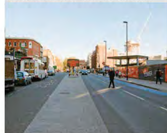
Figure 121: The central median should be paved in the same material as the footway
