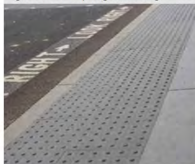
Figure 126: Blister paving at a crossing
