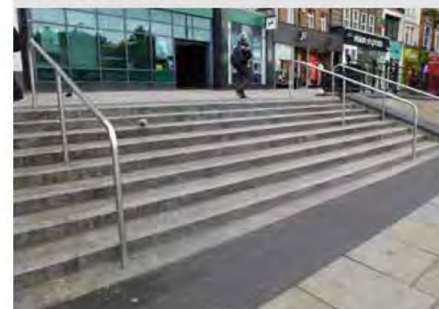
Figure 133: Corduroy paving used at stairs to indicate a level change
