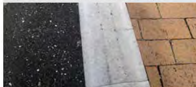
Figure 112: Cycle lane delineator strip
