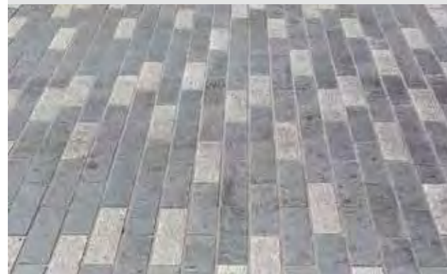
Figure 101: Granite setts used on a carriageway to slow vehicles and create a more pedestrian friendly setting
