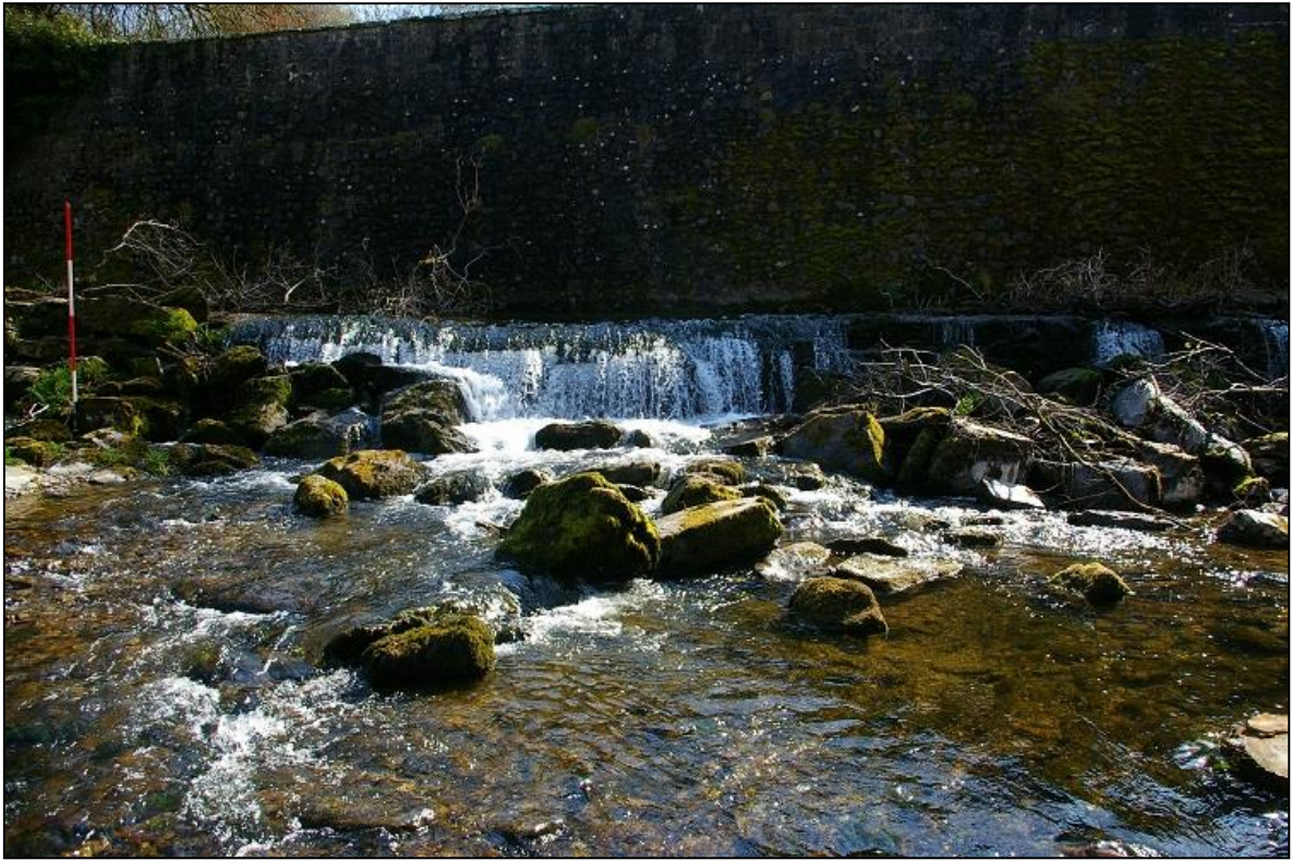
FIGURE 8: THE DROP-WEIR ELEMENT OF THE WEIR, WITH 2M SCALE.
