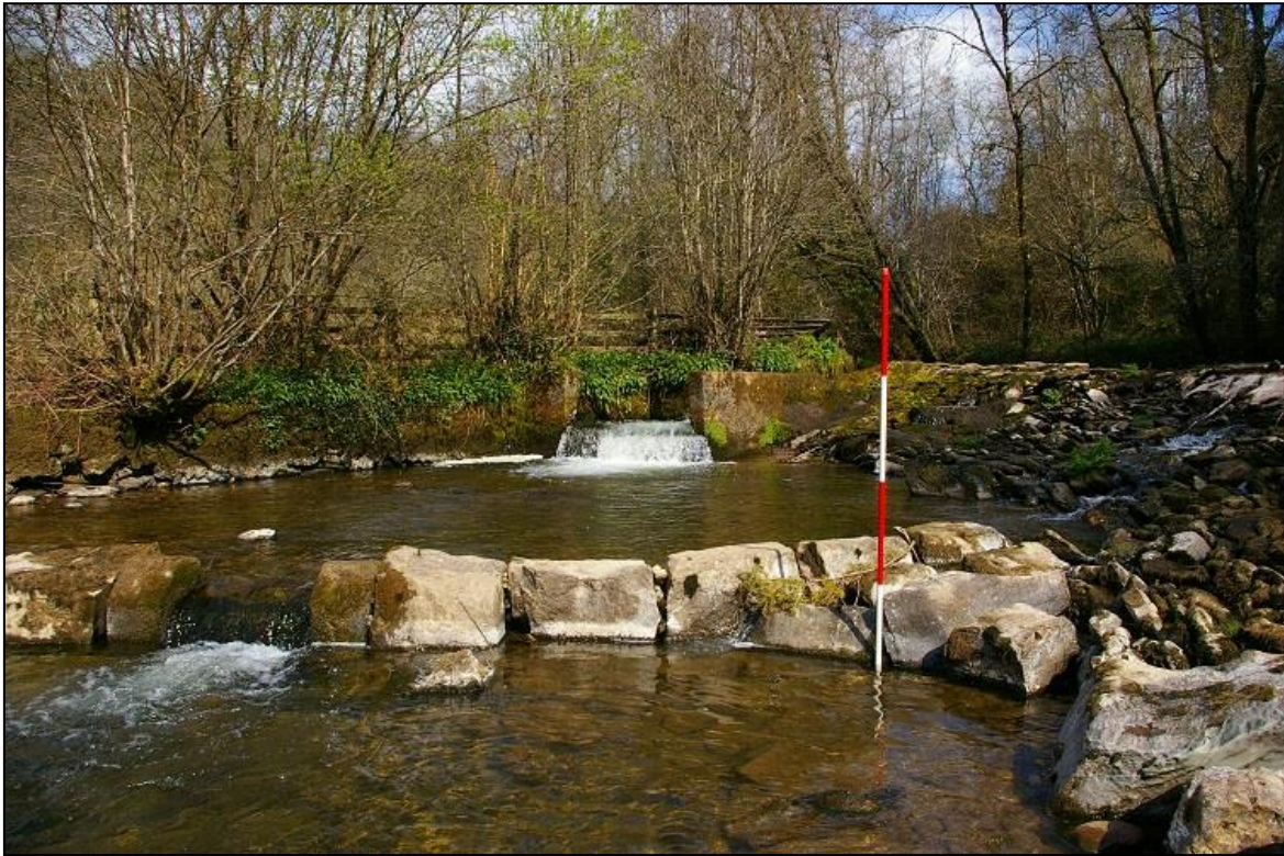
FIGURE 10: THE FISH PASSAGE AT THE NORTH-WEST END OF THE CRUMP SECTION OF THE WEIR, WITH 2012 POOL FORMED IN FRONT, WITH 2M SCALE.
