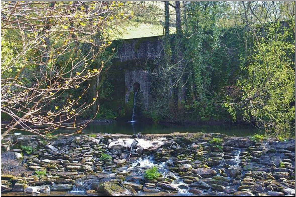
FIGURE 11: THE CULVERT ABOVE THE WEIR, BUILT INTO THE RETAINING WALL ALONGSIDE THE ROAD; FROM THE SOUTH-WEST (NO SCALE).
