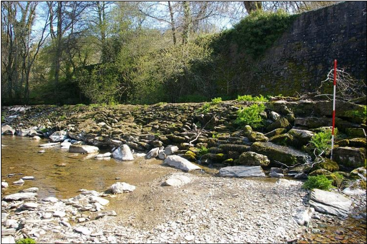
FIGURE 9: THE 'CRUMP' ELEMENT OF THE WEIR, SHOWING LACK OF OVERFLOW; FROM THE SOUTH-WEST (WITH 2M SCALE).
