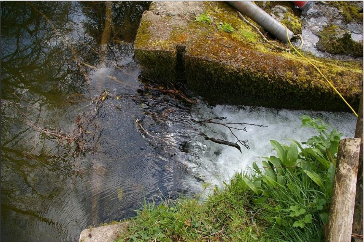
3. VIEW OF THE TOP OF THE FISH PASS WITH SLOTS FOR SLUICE GATE; FROM THE WEST (NO SCALE).
