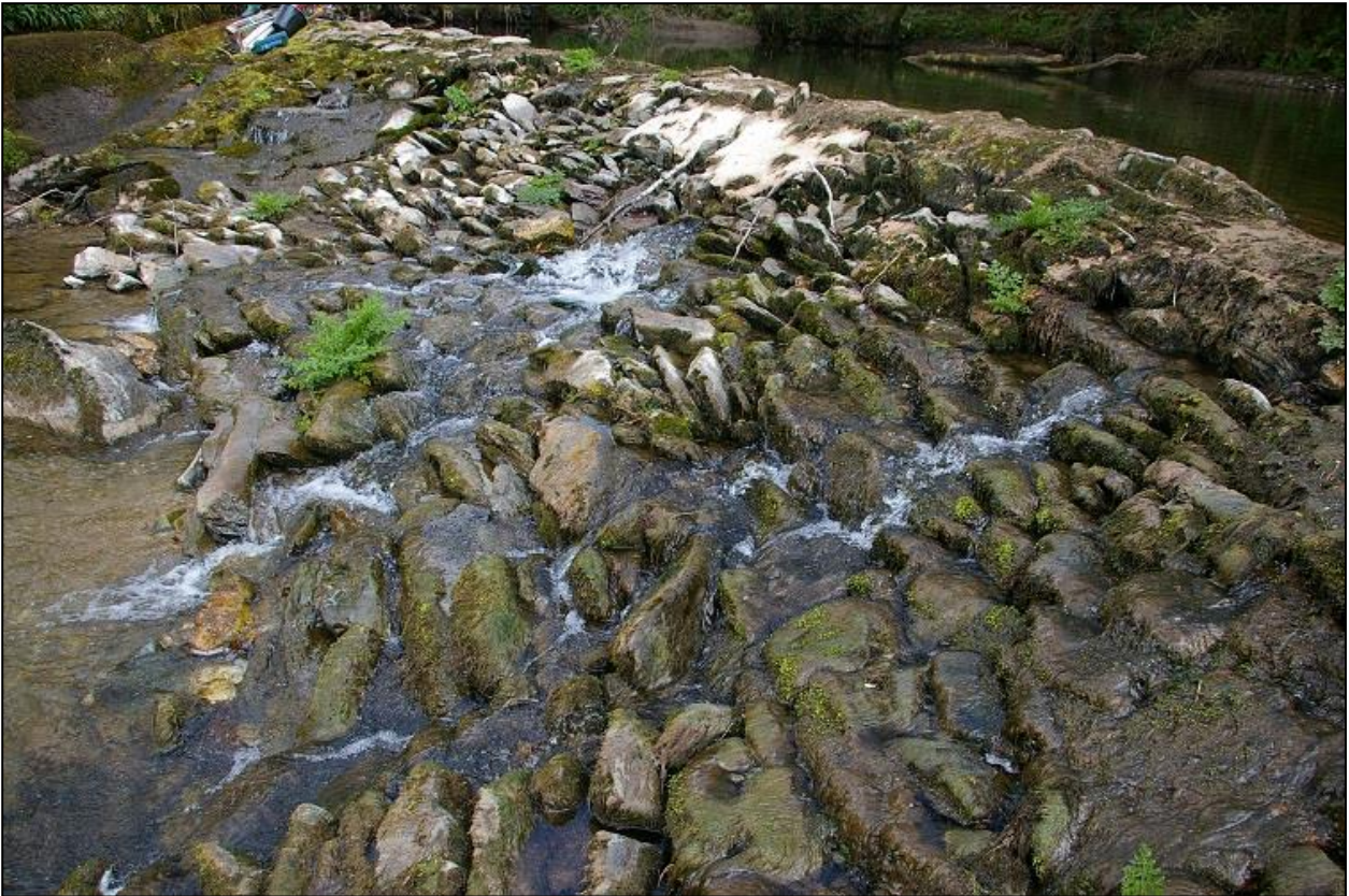
5. DETAILED VIEW OF THE CRUMP STYLE SLOPE, MADE OF LINEAR ARRANGED BOULDERS AND THE SMALL AMOUNT OF WATER WHICH IS OVER-TOPPING THE WEIR; FROM THE SOUTH-EAST (NO SCALE).
